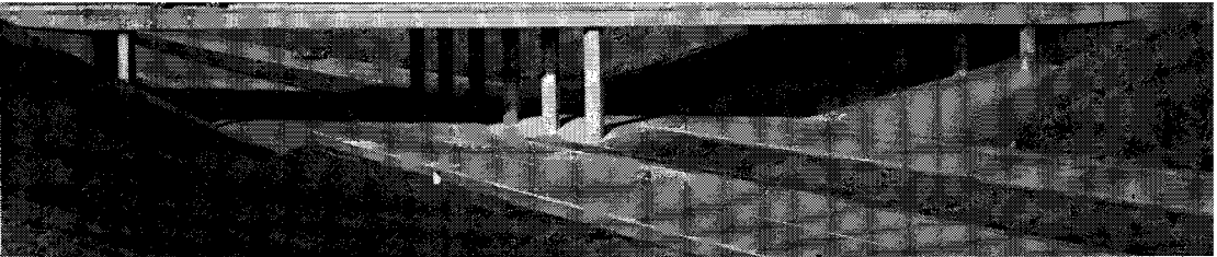
Fig. 1 Slab bridge over Danish turnpike (2 x 20m) with recessed abutments in order to increase visibility on the road.
