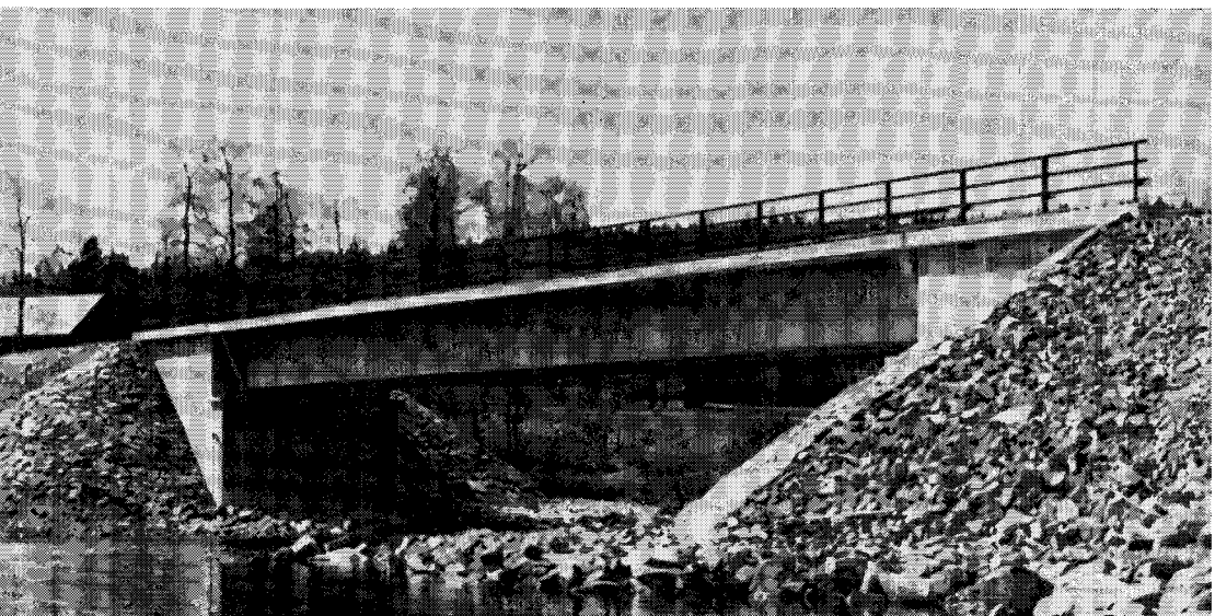
Fig. 2 Simply supported beam bridge over Swedish river (30 m), cast in situ.
