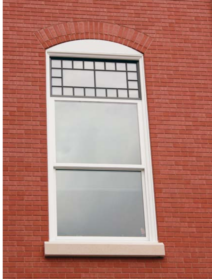
Precast concrete panels in the addition reflect the stately architecture of the original, including matching the brick circa 1890. Photo: Gate Precast Company.
