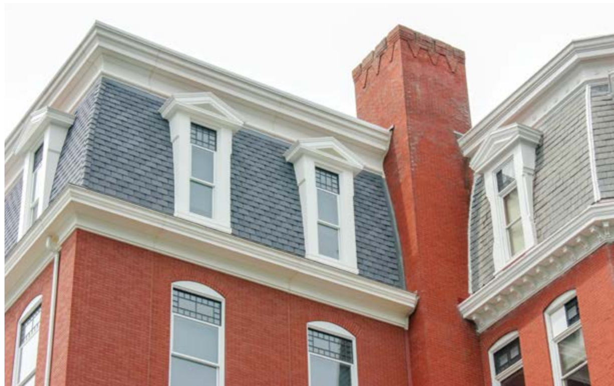
Precast concrete far exceeded expectations in producing an extraordinary level of detail in the panel profile. Photo: Gate Precast Company.
