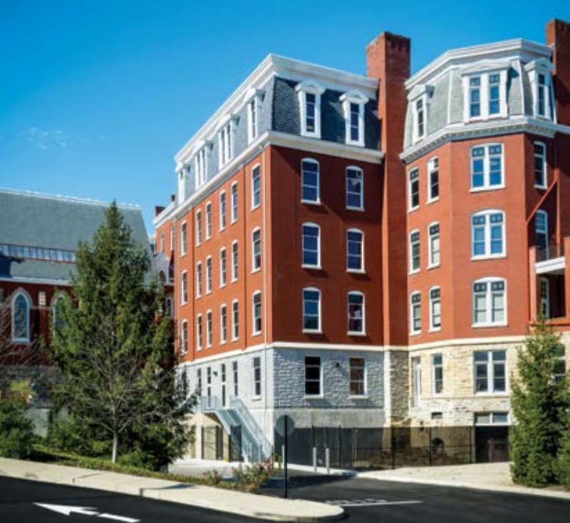
The addition to The Summit Country Day School restored a portion of the structure that had collapsed. The total-precast concrete structure was erected in 22 days. Photo: Joe Harrison, JH Photography Inc.
