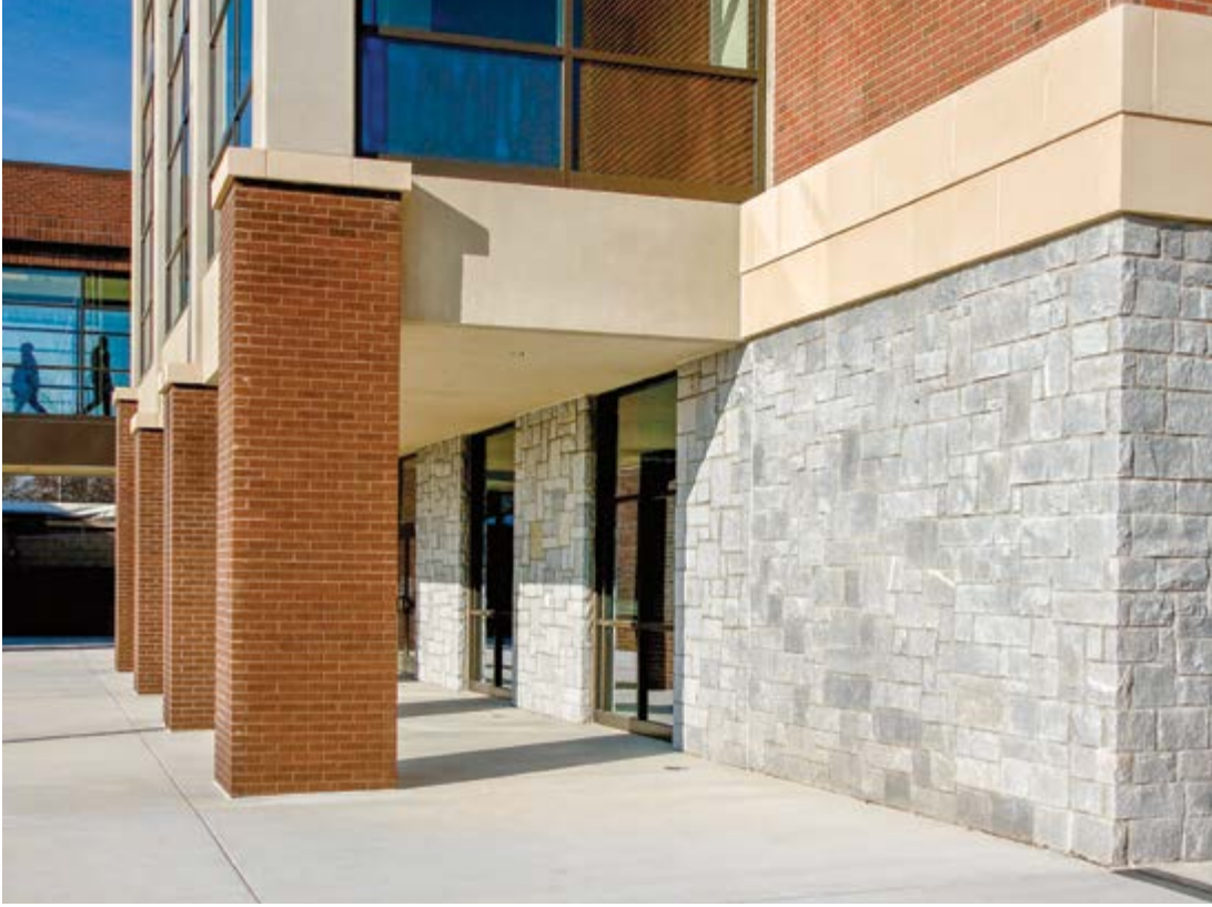
At Tucker High School, the stone veneer at the bottom of the media center is granite hand-set in the precast concrete panels. Photo: George Spence, Metromont Corporation.
