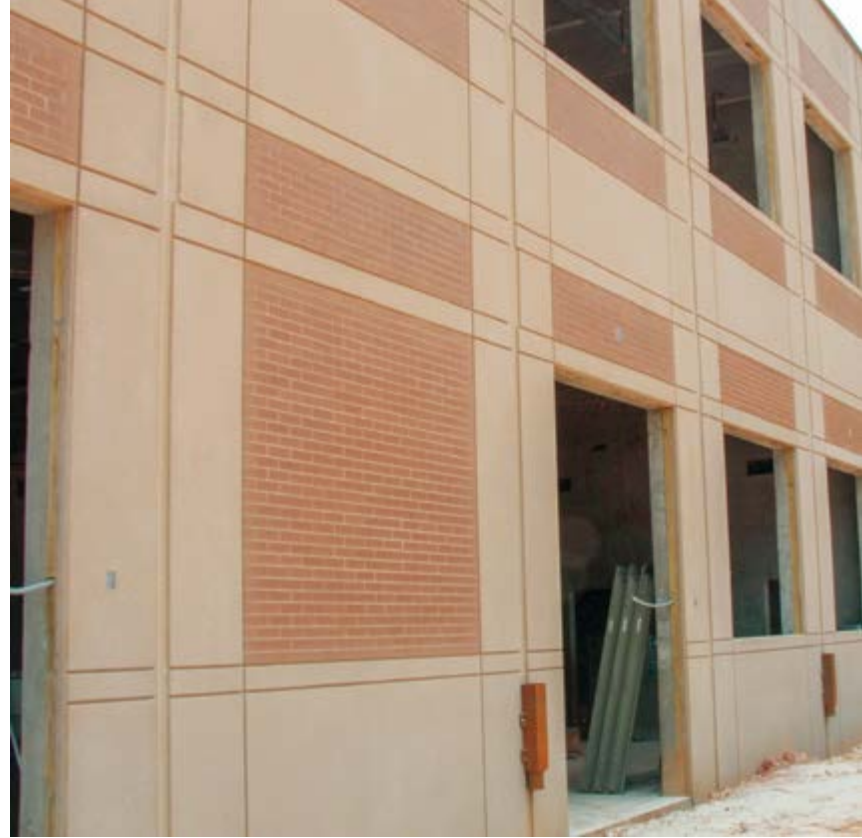
The Eastern Guilford High School design allowed more thin brick to be inset into panels than at Northern Guilford, providing more accents and a warmer appearance.
