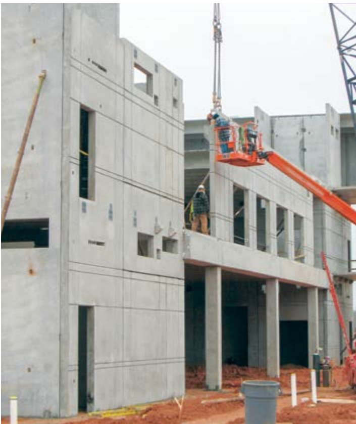
The total–precast concrete structural framing system allowed Eastern Guilford High School to be erected quickly, helping to meet an aggressive schedule after the original building was destroyed. Photo: Tindall Corp.
