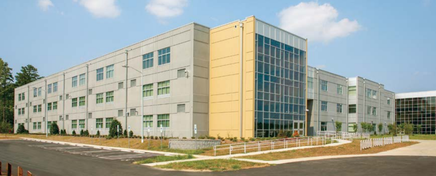
LS3P's design for Ardrey Kell High School served as a prototype for other schools and was reused two years later for the Mallard Creek High School. The 306,000-ft 2 school, which serves 2000 students, features a precast concrete structural system with adaptations to its site.
