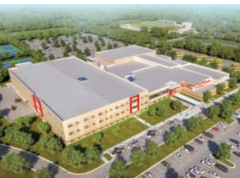
Now under construction, West Cabarrus High School in Concord, N.C., features architectural precast concrete panels and a precast concrete framing system for its classroom sections. Precast concrete’s capability to meet the project’s schedule was a key factor in its specification.
