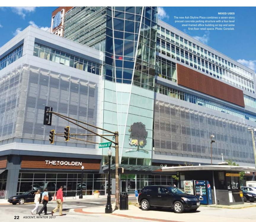
that, the west elevation features an architectural precast concrete fire-separation wall that was designed to be load bearing to accept tees when the project moves ahead.
