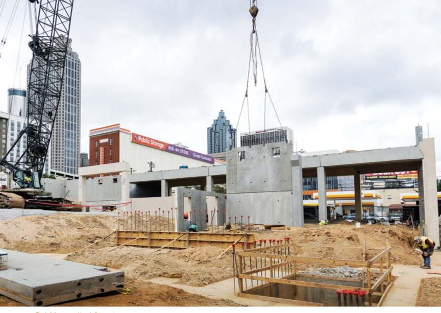
The building, erected in only five months, was completed in phases so interior trades could begin work while the next section was erected. Photo: Metromont.
