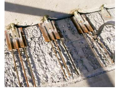
CONNECTIONS Diaphragm to wall connections in University of California–San Diego test building. Photo: PCI.
