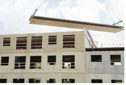
THE FLOOR SYSTEM The floor system offers spans of up to 68 ft, providing open spaces on the first floor while offering needed support for upper-story wall dividers. Photos: Finfrock.
