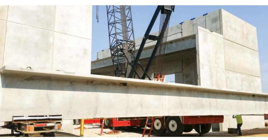
TOTAL-PRECAST A total-precast concrete structural framing system was used to construct most of the performing-arts center at the Kickapoo High School. Photo: Prestressed Casting Co.
