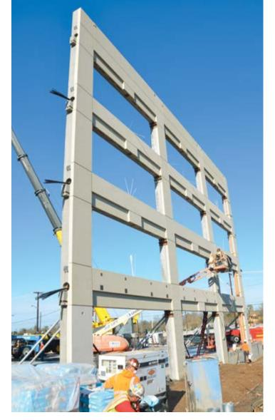
FAST FRAME The entire precast concrete hybrid moment frame system was installed in just 38 days. Photo: Ryan Colditz.
