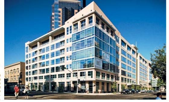
J LOFTS 800 J Lofts was the first total–precast concrete mixed-use structure in California to employ the new precast concrete hybrid moment frame as its chief means of seismic resistance. Photo: LPAS Architecture + Design.
