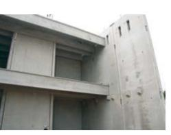
**STRUCTURE FEATURES** The structure features load-bearing precast concrete walls and double tees that rest on haunches built into the panels. Photo: Prestressed Casting Co.
