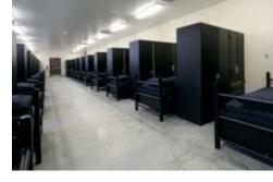
**INTERIOR SPACES** Long-span double tees provided open interior spaces. Walls consist of the interior face of the load-bearing precast concrete panels, which have a smooth troweled finish. Photos: Johnson-McAdams
