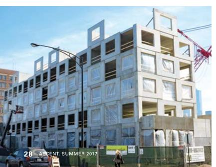
income residential units on this scale. "We definitely needed highquality fireproof construction, and precast concrete met that goal handily," Brown says. It also aided in providing the fire-separation layer required between parking and occupied spaces.
