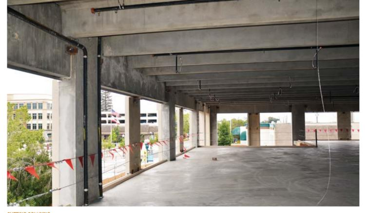
CUTTING COLUMNS The precast design option removed columns and used double tees to create 56-ft spans. Photo: Ryan Colditz.
