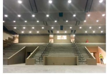
CHALLENGES FOR THE ERECTION OF THE WALL PANELS Precast concrete risers were installed for seating sections, creating challenges for the erection of the wall panels in the tight location. Photo: Prestressed Casting Co.
