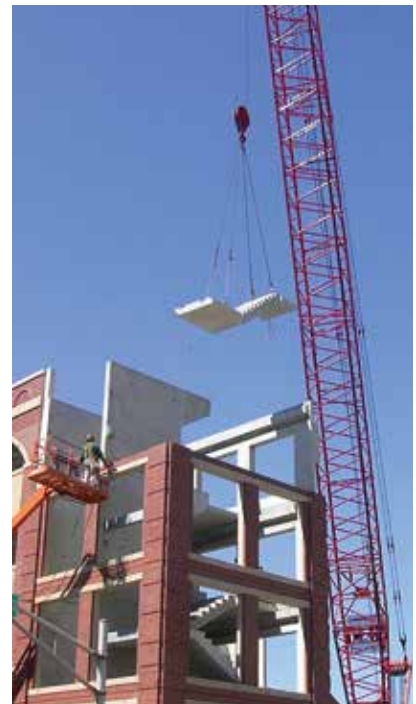
The total-precast concrete structural system provided a quick and easy erection. Many panels feature several finishes, including two colors of thin-set brick and accents. Photos: Rich & Associates.
