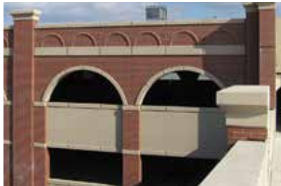
Photo: Coreslab Structures (Indianapolis) Inc.
