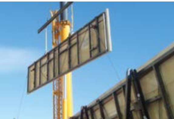
The precast panels, which weigh 30 pounds per square foot, feature a concrete skin attached to a steel frame, with insulation added behind. Photo: Clark Pacific.
