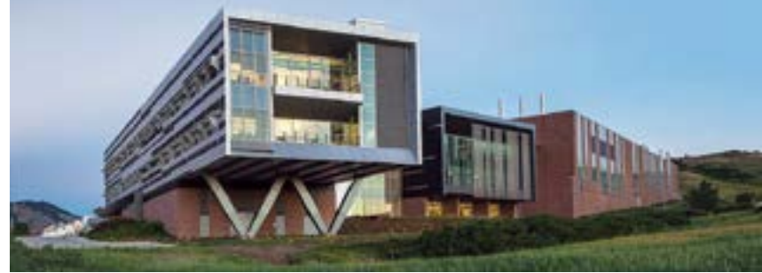
NREL's Energy Systems Integration Facility features Stresscon precast panels insulated with Thermomass System NC to meet both the safety specifications and the energy efficiency demands for the laboratory environment. Photo: U.S. Department of Energy.
