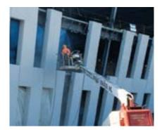
**CUSTOM TOUCH** Each panel on the curved façade required a personal, customized fit to ensure it fit perfectly into its assigned spot. Photo: High Concrete Group.
