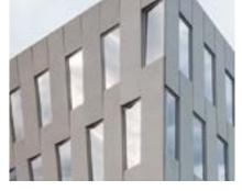
TIGHT CORNERS Only the front façade curves, creating challenges in matching its design to the three flat sides. Photo: High Concrete Group.
