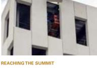
Shorter, square panels were used to finish off the alternating pattern of panels at the roofline. Photo: High Concrete Group.
