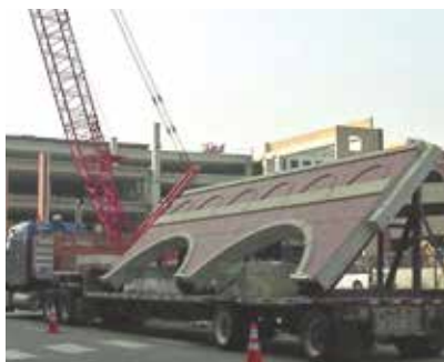
The total-precast concrete structural system provided a quick and easy erection. Many panels feature several finishes, including two colors of thin-set brick and accents. Photos: Rich & Associates.
