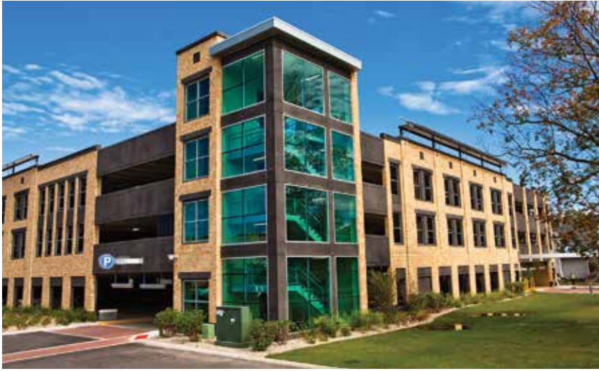
The Old Town Parking Structure in Traverse City, Mich., features a variety of sustainable-design concepts generated from public design charrettes. These include a green roof over a portion of the roof-level parking and atop the stair towers, charging stations for electric vehicles, solar panels to generate electricity, and a snow-melt system.
