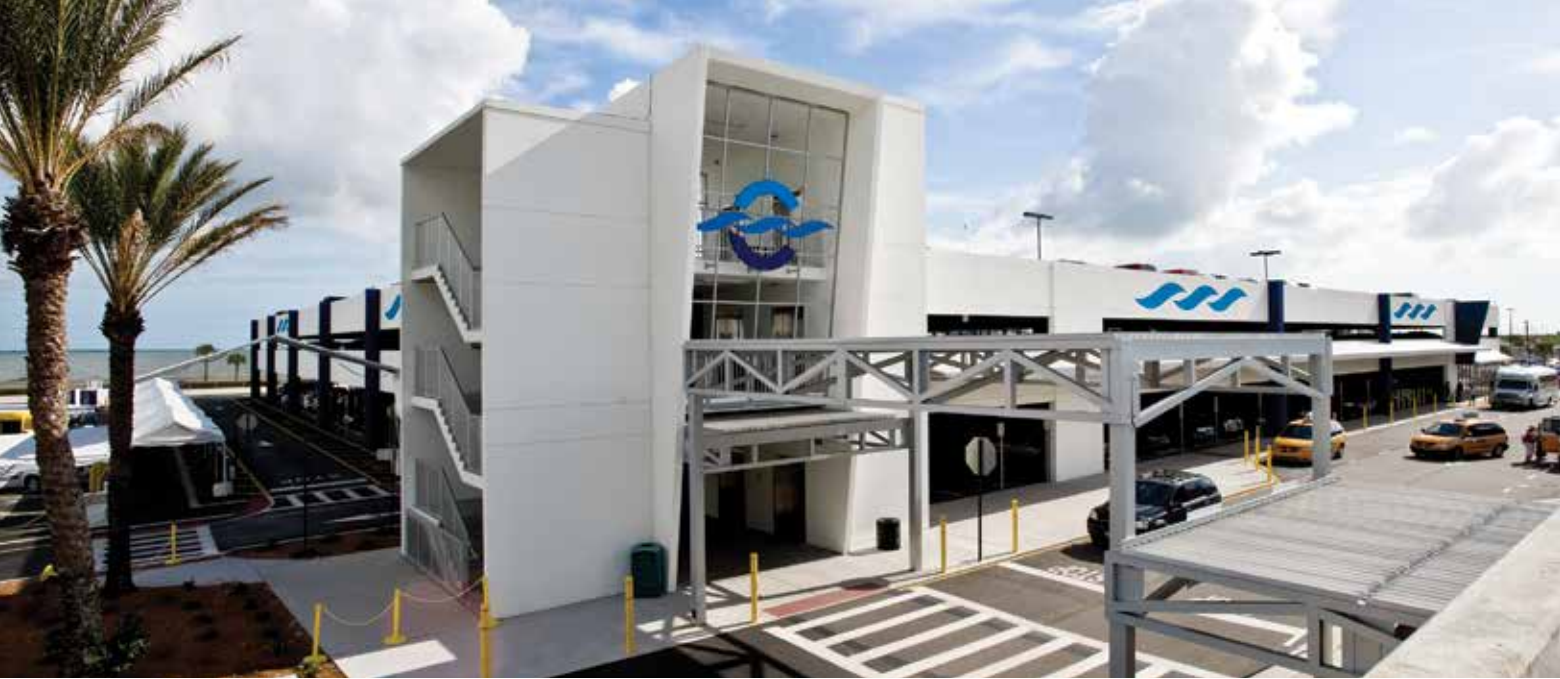
Precast concrete spandrels had the terminal's blue logo cast into them, after which they were painted to create a dimensional appearance. Photo: Finfrock.
