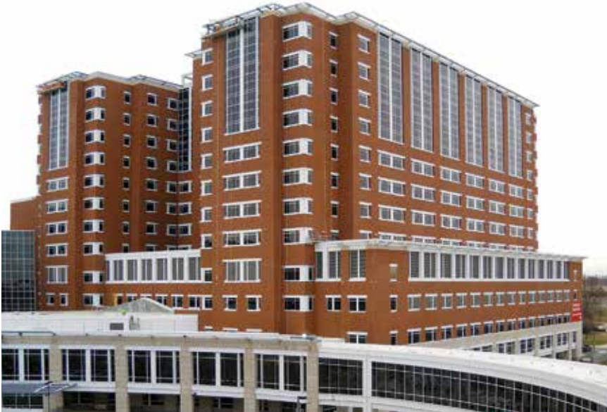
Gate Precast teamed with Thermomass to provide insulated architectural precast cladding panels for the Chandler Hospital Pavilion at the University of Kentucky.
