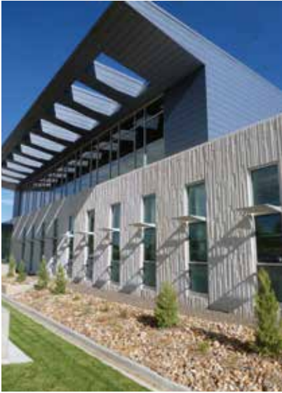
Thermomass-insulated precast panels from Stresscon help reduce energy costs while maximizing interior space for the recent Loveland Service Center project.
