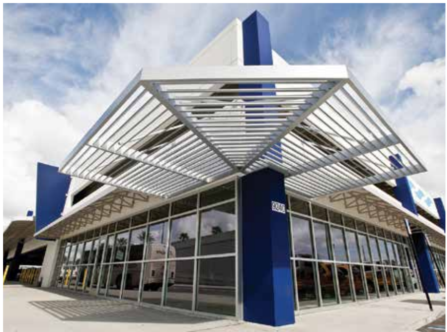
Design-build packages are typically used for the parking structures, allowing bidders to use their most innovative techniques and custom expertise to create the most efficient system. Photo: Finfrock.
