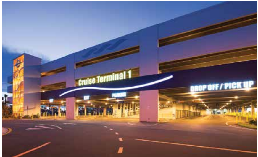
Cruise Terminal, which was recently completed, features passenger drop-off and baggage-handling services on the first level, with parking spaces on the second floor up. The 433,764-square-foot project was constructed, along with the new terminal, in less than 12 months to serve the Royal Caribbean line. Photo: Finrock.
