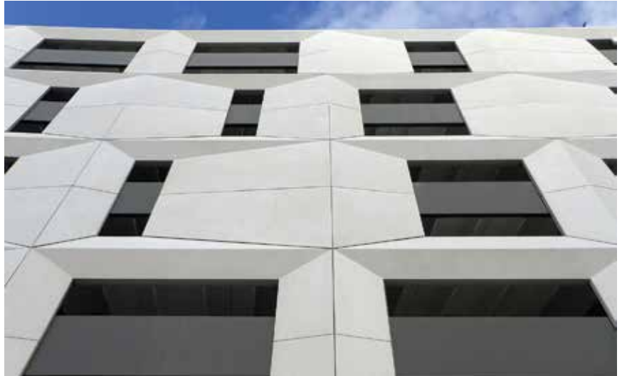
The Z, a 10-story, 1,282-car parking structure creates a "parking experience" for users of a nearby mixed-use building designed to revitalize the district. The precast concrete façade features trapezoid-shaped spandrels that create large, dimensional windows along its length and horizontal openings that band the structure. All photos: Rich & Associates.
