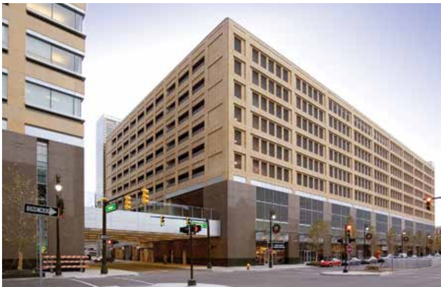
The Campus Martius One parking structure in Detroit, Mich., was value-engineered from cast-in-place to precast concrete to provide a more efficient design. The nine-story, 2,100-car structure features a façade clad with Mankato limestone to match a nearby office building and 16,000 square feet of ground-floor retail space.
