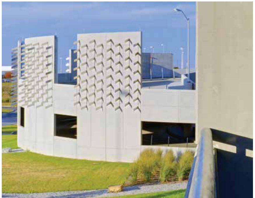
The precast concrete system at the Nashville CON-RAC facility provided a variety of dramatic elements, including a curved helix-ramp enclosure to which sculptural pieces were attached (below). Photos: Demattei Wong Architecture
