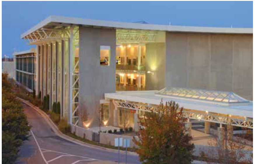
The CONRAC facility at Nashville International Airport features a total precast concrete structural system, which met designers' goals for efficiency, aesthetics, economics, and sustainable design, among others. The three-level facility houses space for 2,400 rental cars along with related services. Photo: Demattei Wong Architecture.
