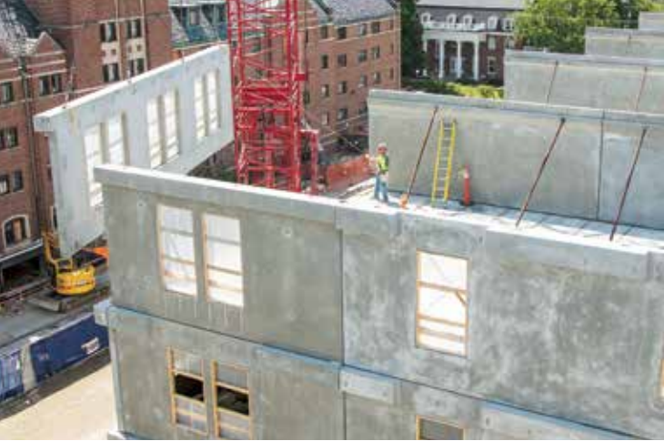
The precast concrete system features architectural precast concrete wall panels, hollow-core floors, stairs, stair walls, interior demising walls, and other components.
