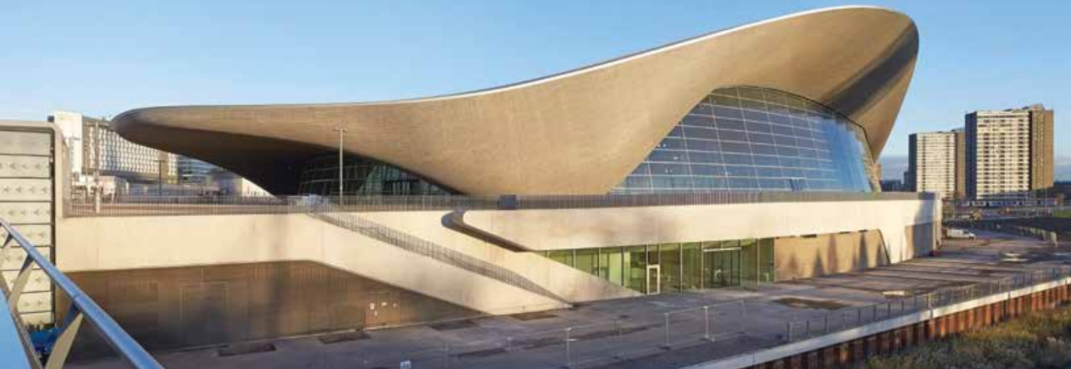
The concrete surfaces on Hadid's Aquatics Centre in London, England, designed for the 2012 Olympic Games, were left exposed to use the texture and finish as a design statement. Photo: ©Hufion+Crow.
