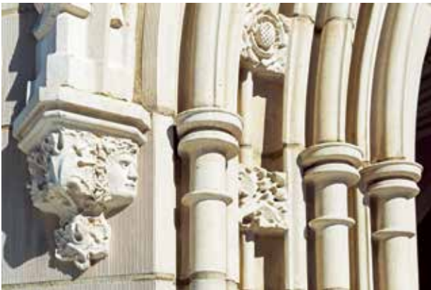
Many of the pieces were quite elaborate and required sculpting of a new piece that then was used to create molds for casting.
