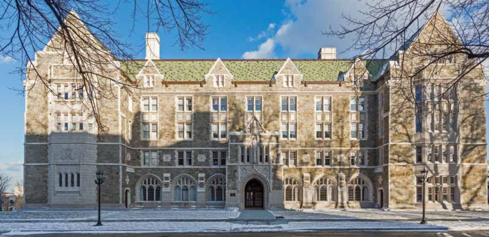
St. Mary's Hall at Boston College, Chestnut Hill, Mass., used more than 15,000 pieces of precast concrete to replicate the look of the cast stone originally used to clad the building, constructed in 1917.
