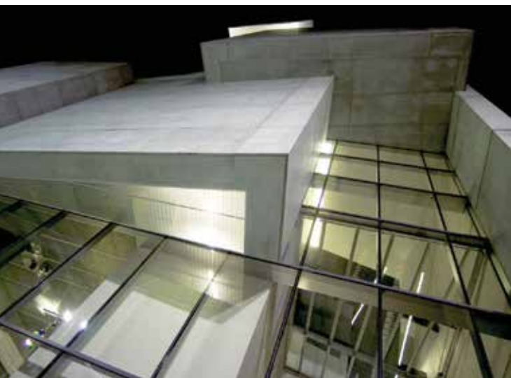
The Rosenthal Center for Contemporary Art in Cincinnati, Ohio, built in 2003, features a dramatic “as-cast” finish to emphasize the raw concrete material. The New York Times called it “the most important new building in America since the Cold War.”
