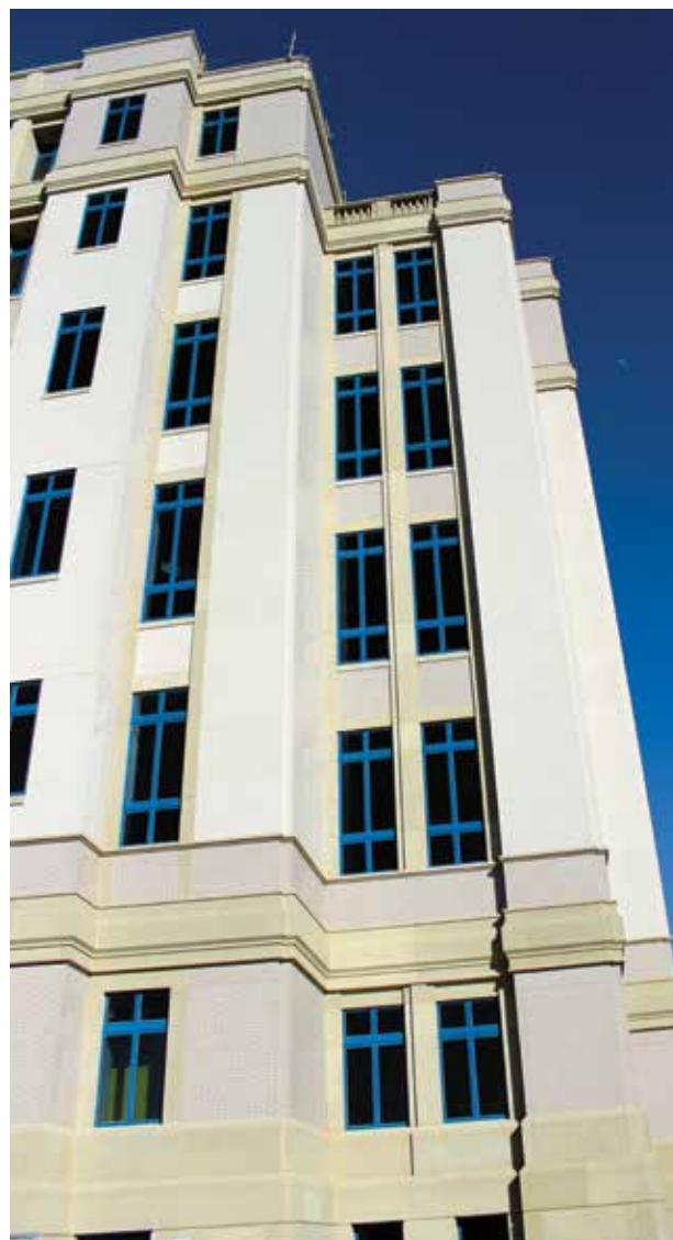
Gate used a new chemical process to create an appearance that emphasized the random coloring and veining of actual stone.
