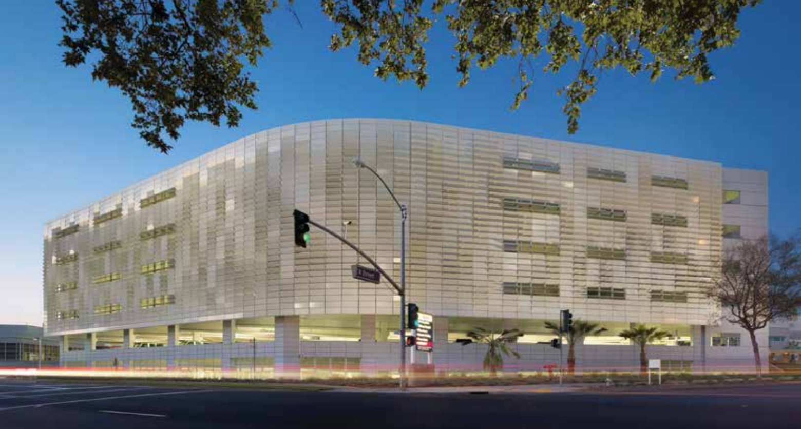
The new six-level, 400,000-square-foot parking structure at the gateway to the University of California at Davis Medical Center in Sacramento, Calif., features a precast concrete hybrid moment frame that allows the structure to self-right after a seismic event. A distinctive “lap-siding” design for spandrels provides visual interest while helping to keep the façade clean.
