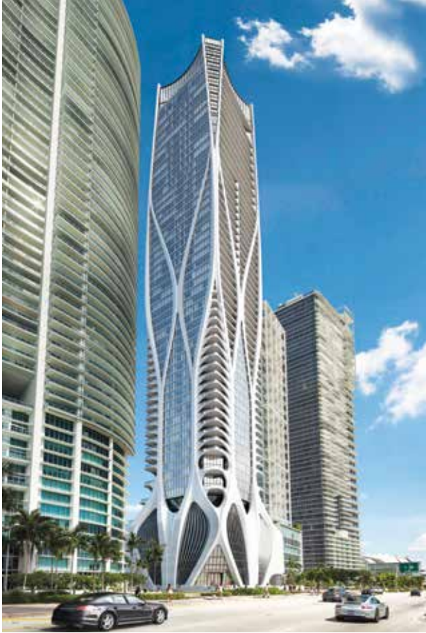
The 1000 Museum condominium project in Miami, Fla., currently under construction, features an exoskeleton of GFRC panels being shipped from Dubai by a PCI-certified precaster. The design provides a rigid exterior frame that will be functional and decorative. Rendering: © 2014 Paul Morris.
