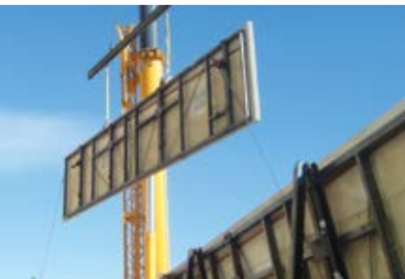
The precast panels, which weigh 30 pounds per square foot, feature a concrete skin attached to a steel frame, with insulation added behind. Photo: Clark Pacific.
