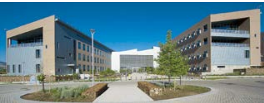
Rocky Mountain Prestress teamed with Thermomass to provide durable insulated panels to protect the NREL Research Support Facility from all manner of Colorado weather while also forming an integral piece of the building's passive heating and cooling operations. Photo: U.S. Department of Energy.
