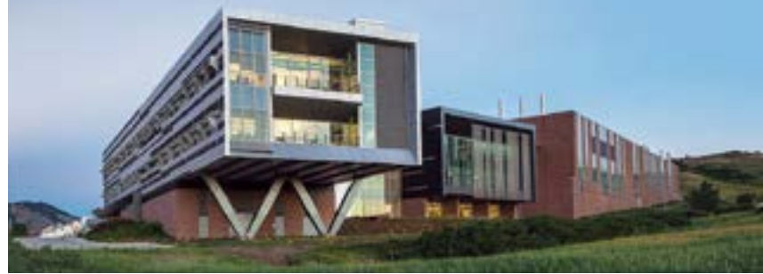
NREL's Energy Systems Integration Facility features Stresscon precast panels insulated with Thermomass System NC to meet both the safety specifications and the energy efficiency demands for the laboratory environment. Photo: U.S. Department of Energy.
