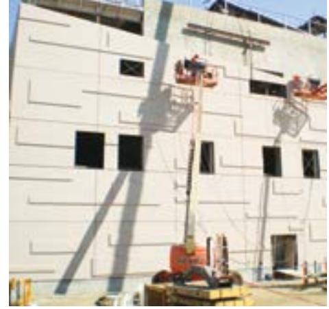
The panels were cast and delivered to the site for immediate erection as the schedule required, eliminating site congestion. Photo: Clark Pacific.
