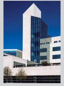
The new Martin Army Community Hospital features precast concrete in the exterior skin and the sandwich panels of the main structure. There are also two total precast parking decks built as a part of this project.
