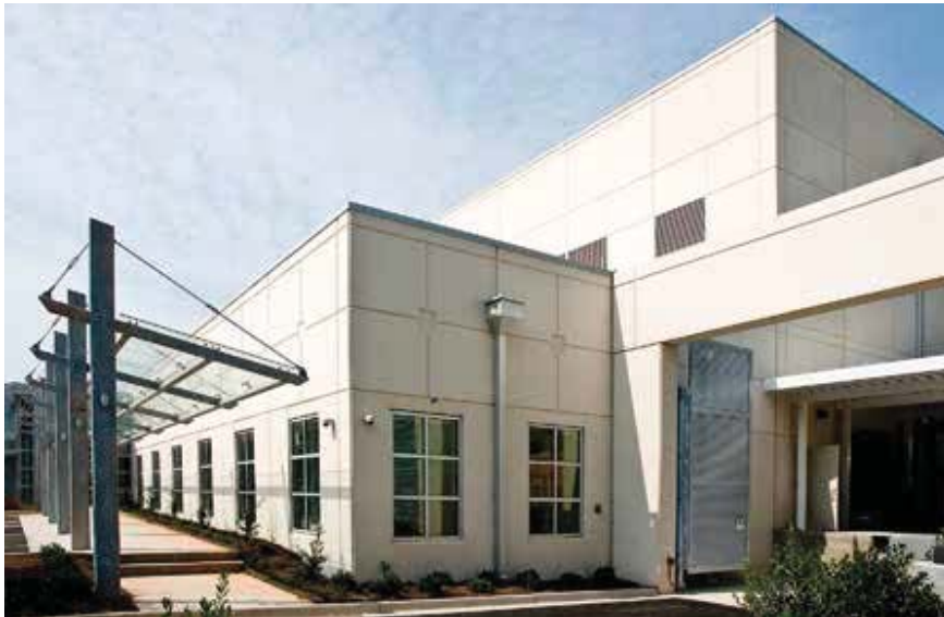
The precast concrete panels cladding the building were typically 12 feet wide and 37 feet tall, with blockouts for ventilations ducts and other HVAC needs added on the second level. Photo: Metromont Corp.
