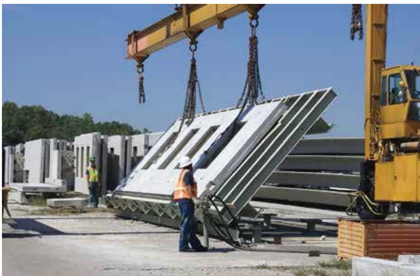
First-floor panels features a variety of windows cast into the panels, with interior insulation running up against the penetrations. Photo: Metromont Corp.
