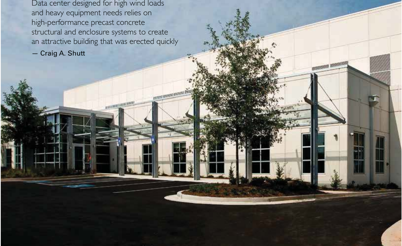
A data center in Georgia took full advantage of the benefits provided by a high-performance precast concrete structural and enclosure system to gain enhanced impact resistance, thermal efficiency, and other specialized features. Photo: Metromont Corp.
