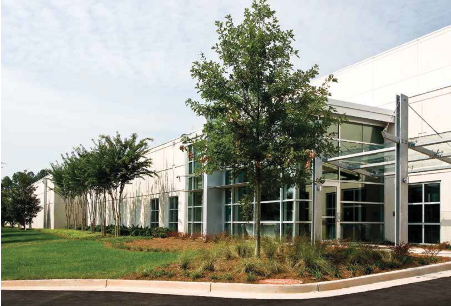
The building's first floor features offices, while the processing equipment was placed on the second floor, with no windows interrupting the panels. Photo: Metromont Corp.
