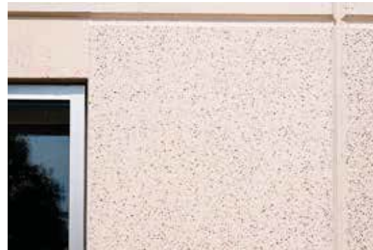
The panels feature an off-white face mix with a light sandblasted finish, which matched the finish on the original building erected four years earlier by the same design and construction team. Photo: Metromont Corp.
