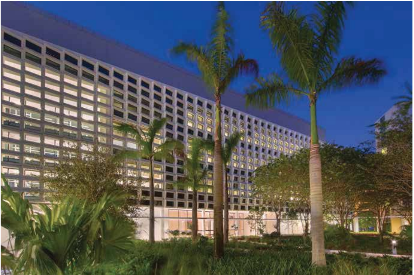
Precast concrete panels with integrated window units were used on the six-story Science Classroom Complex at Florida International University. The project was done on a design-assist basis, allowing the precaster to work with subcontractors during the design process to integrate as many materials as possible. Photo: Gate Precast Co.
