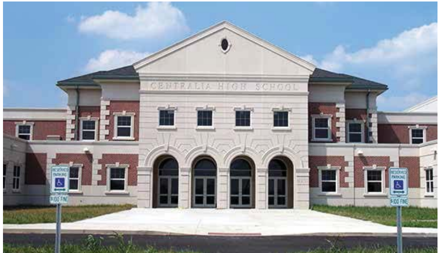
Designers for Centralia High School in Centralia, Ill., specified embedded thin brick on precast concrete insulated sandwich panels and also integrated electrical conduit and boxes. Casting in those services at the plant saved considerable time at the site and reduced trade congestion. Photo: Gate Precast Co.
