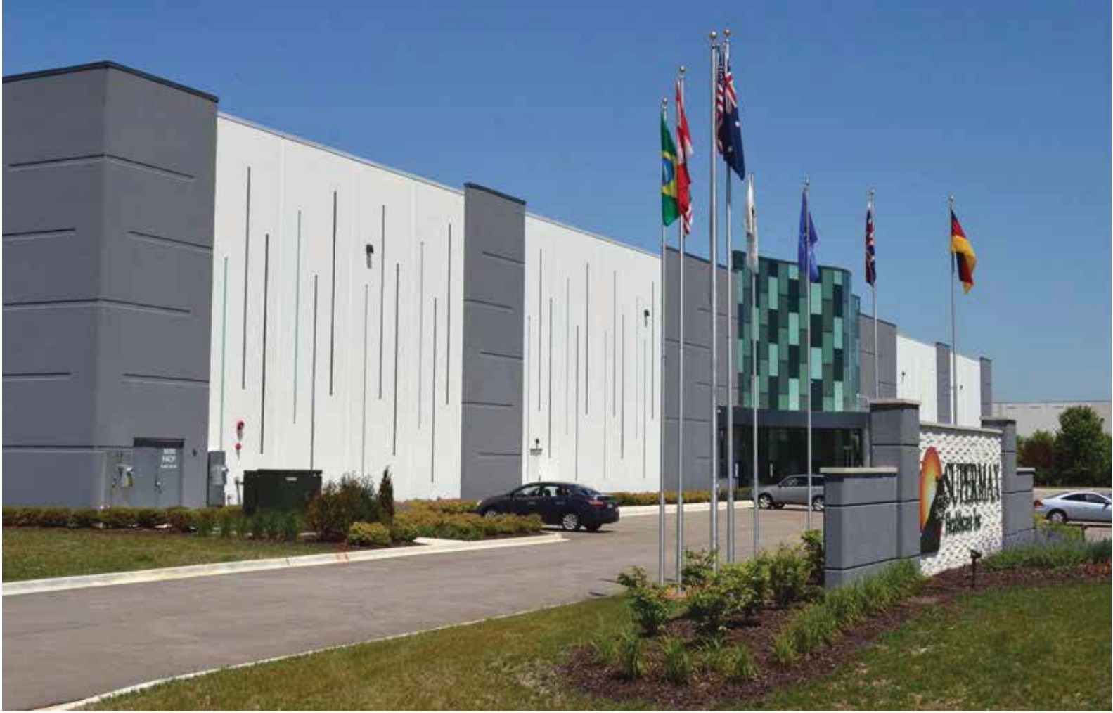
The 90,170-square-foot SuperMax Distribution Center in Aurora, Ill., features insulated precast concrete panels that helped the facility achieve a Gold LEED rating. Photos: ATMI Precast.
