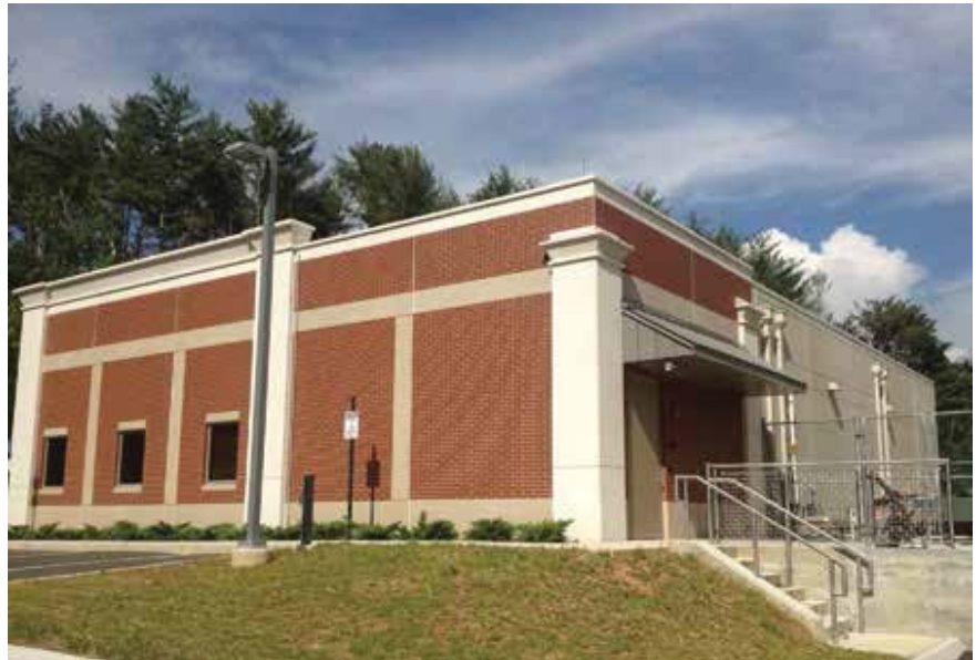
The 4,500-square-foot Tier II+ data center at Washington & Lee University required a tight schedule to ensure funding remained available for the project. Load-bearing architectural precast concrete insulated sandwich wall panels and hollow-core slab helped to meet a variety of challenges in completing the project. Top Photo: Hoch Associates. Others: Gate Precast Co.
