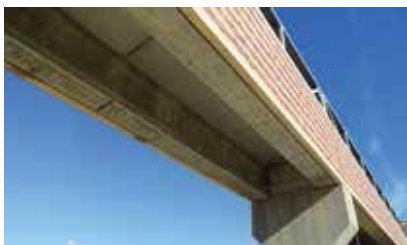
Three separate buildings, including a one-story parking structure built with a total-precast concrete structural system, created a state-of-the-art bus facility for the Washington Metropolitan Area Transit Authority in Washington, D.C. The three facilities were clad with architectural precast concrete panels embedded with thin brick to create a consistent and attractive appearance. Photos: Shockey Precast Group.
