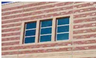
Three separate buildings, including a one-story parking structure built with a total-precast concrete structural system, created a state-of-the-art bus facility for the Washington Metropolitan Area Transit Authority in Washington, D.C. The three facilities were clad with architectural precast concrete panels embedded with thin brick to create a consistent and attractive appearance. Photos: Shockey Precast Group.
