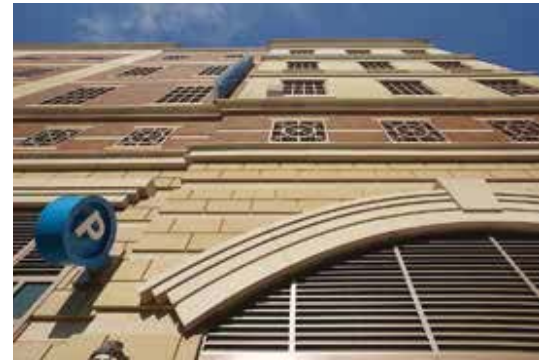
A historic-like appearance was created for the architectural precast concrete panels cladding the 151,200-square-foot Lancaster Newspaper Parking Garage in Lancaster, Pa. The look had to be approved by the city's Historical Architectural Review Board. The structure consists of a total-precast concrete structural framing system. Photo: Nathan Cox Photography.
