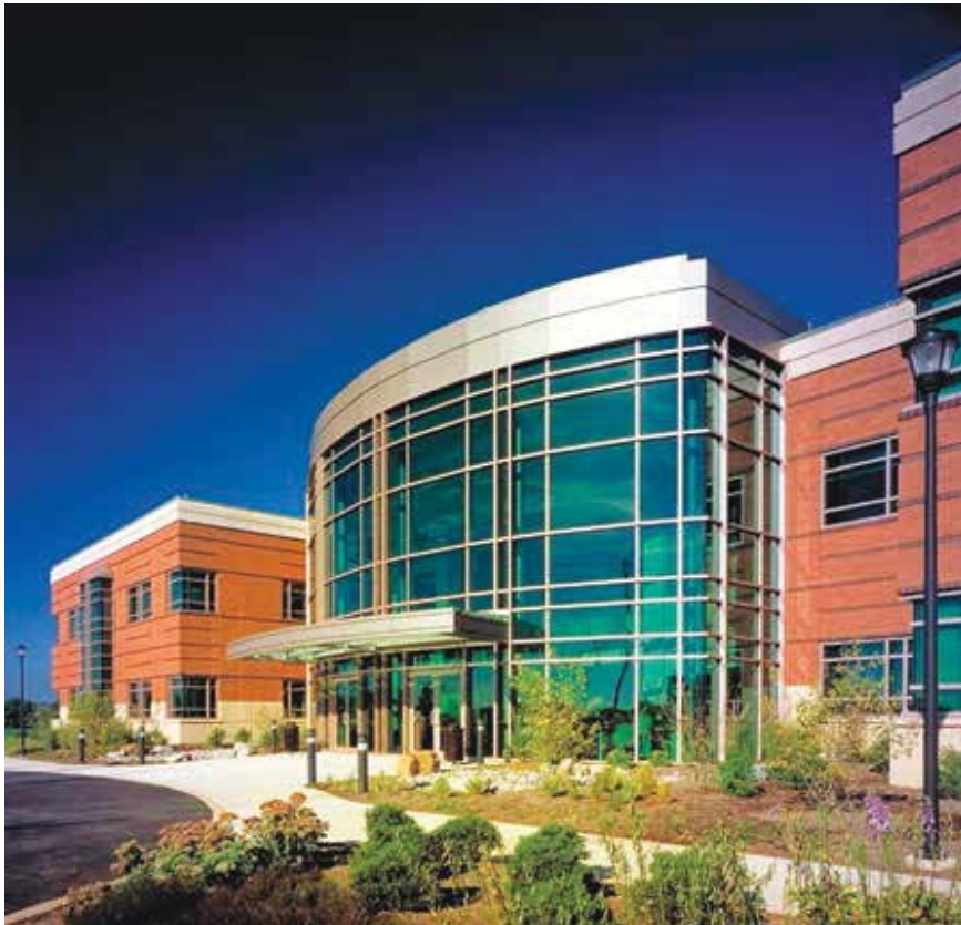
The 146,000-square-foot Bosch Security System manufacturing building in Lancaster, Pa., features architectural precast concrete panels, while the 66,000-square-foot, two-story office building next door offers a mix of precast concrete and hand-laid brick. A glass corridor connects to two, allowing them to be separated when sold if needed. Photo: Terry Corbett Photography.
