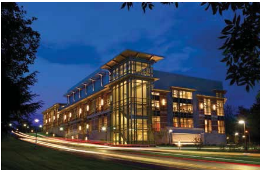
The new addition to the Messiah College Performing Arts Center in Mechanicsburg, Pa., was clad with precast concrete panels faced with cast-stone pieces. The project was complicated by its steeply sloping site and the need to maintain occupancy of the existing building during construction. Photo: Nathan Cox Photography.
