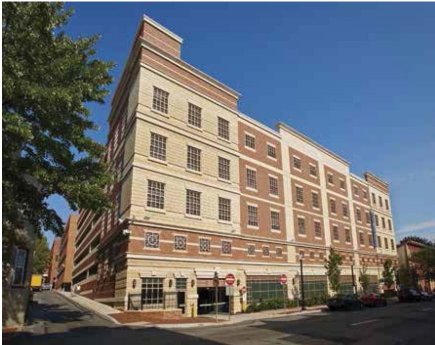
A historic-like appearance was created for the architectural precast concrete panels cladding the 151,200-square-foot Lancaster Newspaper Parking Garage in Lancaster, Pa. The look had to be approved by the city's Historical Architectural Review Board. The structure consists of a total-precast concrete structural framing system. Photo: Nathan Cox Photography.
