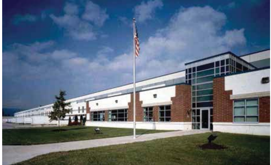
One of Frank Fox's first projects at Greenfield Architects involved designing a Sherwin-Williams distribution center, which featured architectural precast concrete panels with a variety of textures and details. Photo: CB Verlund Photography.
