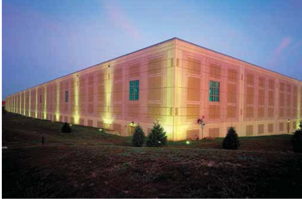
The owners of the new prosciutto-processing plant in Freeland, Pa., requested a total-precast concrete structural system for the project from the beginning, recognizing the benefits that the system can provide to specialized food-processing facilities. Photo: Greenfield Architects.
