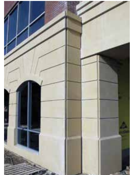
A 40-year-old rundown, vacant building in Summit, N.J., was transformed into a Class A office building by demolishing the structure to its original concrete core, adding a 30,000-square-foot addition and cladding the entire new frame with architectural precast concrete panels. All photos: US Concrete Precast Group.
