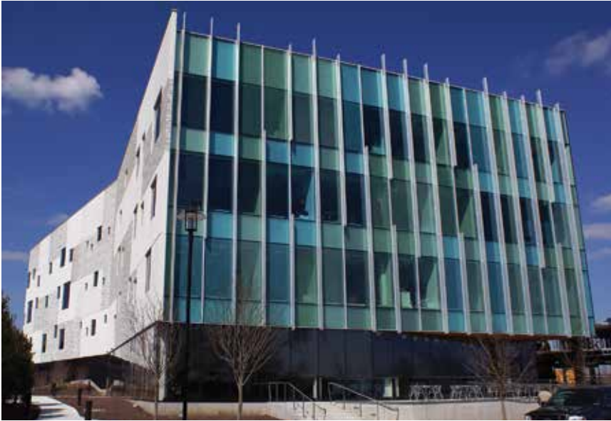
The Iroko Building in Philadelphia was built on a tight time frame so a growing pharmaceutical company could expand its operations. The precast concrete panels used to clad the building helped speed up construction, meet the aesthetic challenges, and help attain LEED certification. All photos: Dave Thomas.
