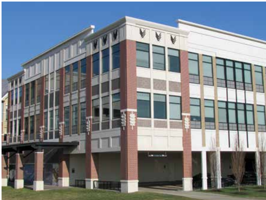
Park Place in Leawood, Kan., used architectural precast concrete panels in different design styles to complement yet differentiate two new buildings in a large upscale mixed-use complex consisting of retail, restaurant, residential, and office spaces. Schedule and aesthetics were key drivers for selecting precast concrete panels. All photos: Dirk McClure of Enterprise Precast Concrete, Inc.
