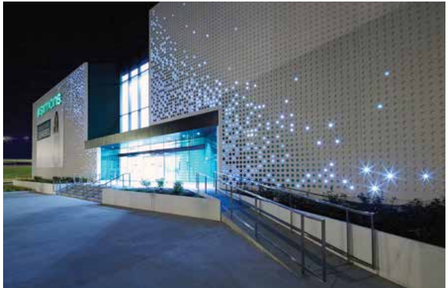
La Maison Simons in Ville d’Anjou, Quebec features architectural precast concrete panels cast with a regular pattern of varying-depth recessed dots fit with fiber optics that illuminate colored disks inside the recesses, changing the look of the building during the day and night. All photos: ©Marc Cramer.
