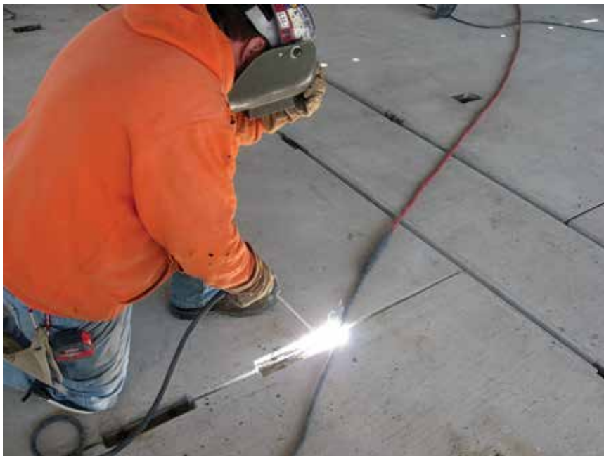
Stainless weld connections and proper precast joint alignment.
