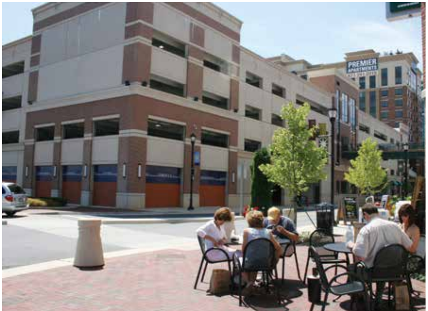
The Annapolis Towne Centre Garage provides dedicated spaces that help support the wide variety of uses for the facility, including banking, retail, condominiums, apartments, luxury hotel, fitness center, office space, and restaurants. Photo: TimHaahs.
