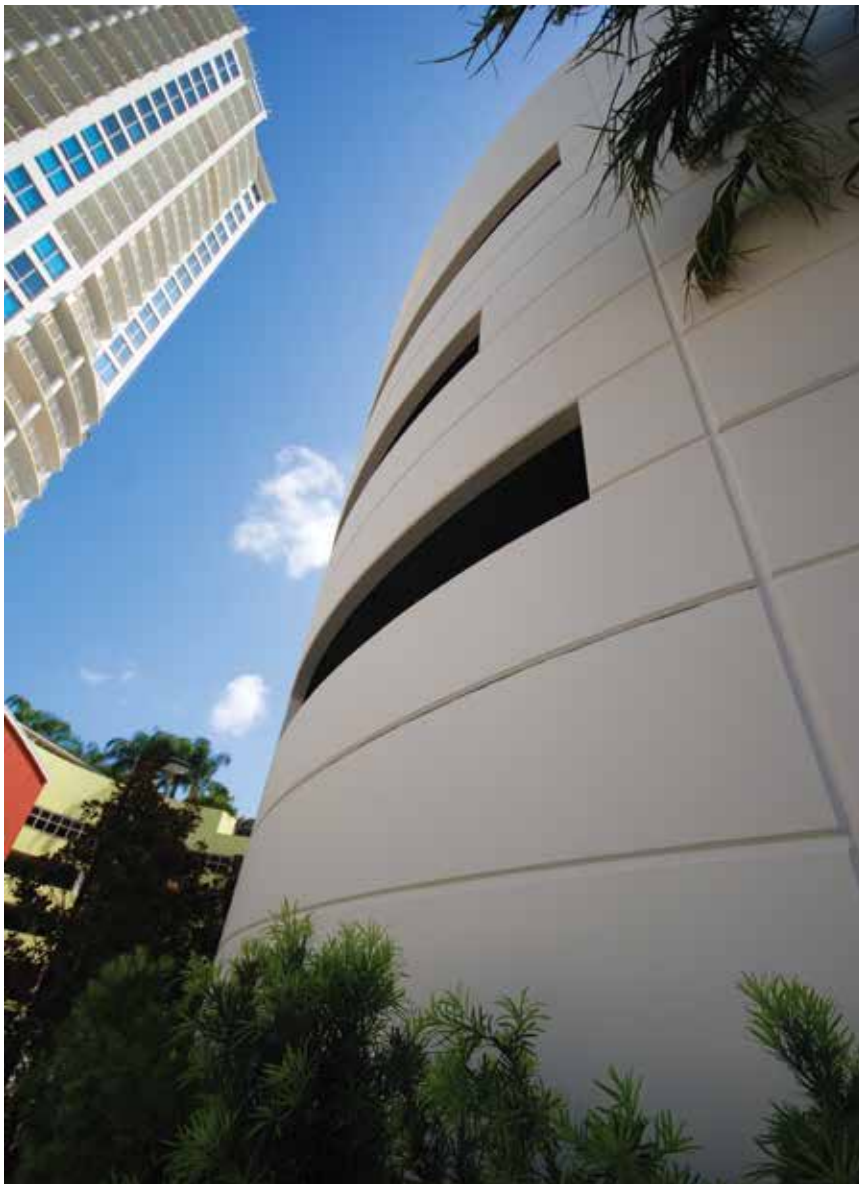
High performance and durability were requirements for the Channelside District parking structure in Tampa, Fla., situated along a Tampa Bay inlet. The facility was designed to encourage more visitors to come to the popular dining and entertainment district.
