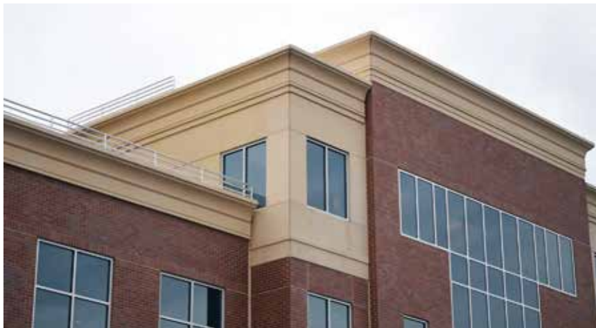
A 40-year-old rundown, vacant building in Summit, N.J., was transformed into a Class A office building by demolishing the structure to its original concrete core, adding a 30,000-square-foot addition and cladding the entire new frame with architectural precast concrete panels. All photos: US Concrete Precast Group.
