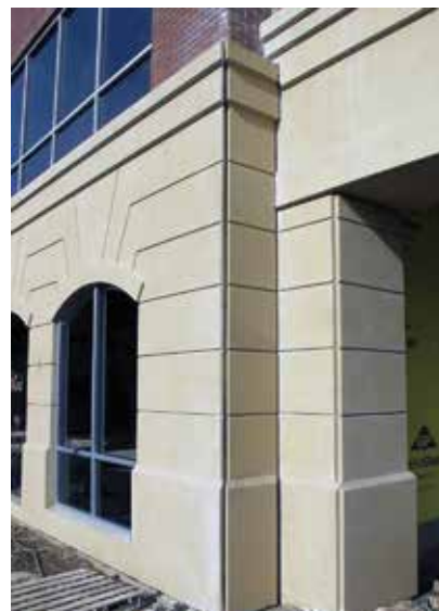
A 40-year-old rundown, vacant building in Summit, N.J., was transformed into a Class A office building by demolishing the structure to its original concrete core, adding a 30,000-square-foot addition and cladding the entire new frame with architectural precast concrete panels. All photos: US Concrete Precast Group.
