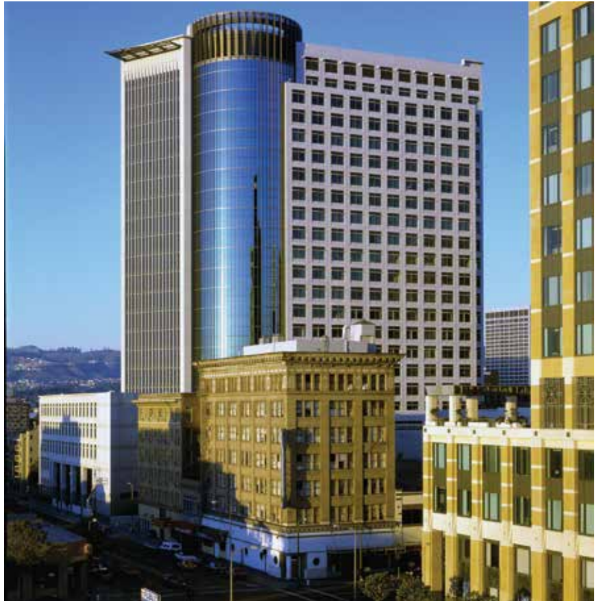
The 22-story tower on the Elihu M. Harris State Office Building in Oakland features inset windows framed by precast concrete pilasters to blend with the architectural character of the neighborhood. Upper stories are clad in textured precast concrete panels. Photo: Nick Merrick, Hedrich Blessing
