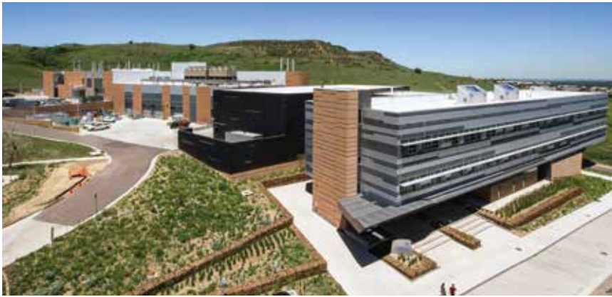
The Energy System Integration Facility in Golden, Colorado used high performance precast concrete to help meet their Net Zero goals. Photo: Dennis Schroeder, NREL.
