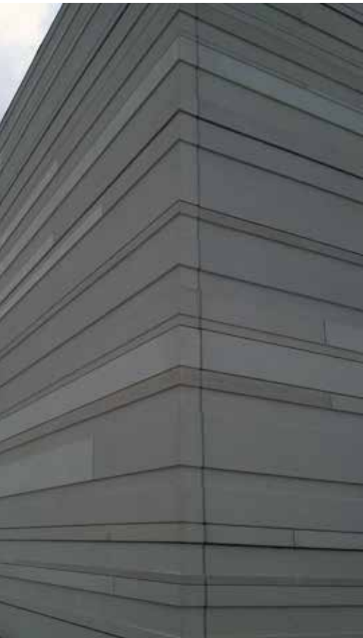
The panels feature 2 or 3 inches of rigid continuous insulation sandwiched between two wythes of precast concrete. Photo: Gage Brothers Concrete Products.
