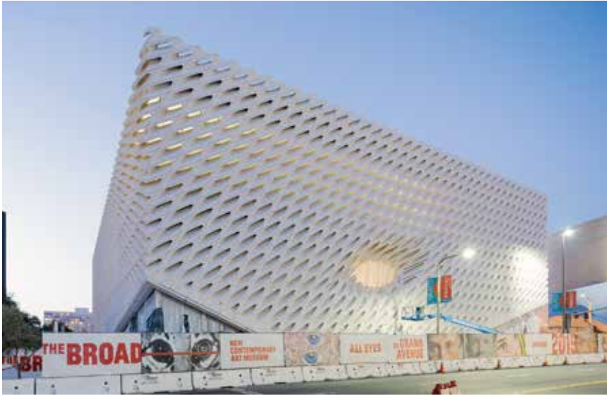
The Broad contemporary art museum in Los Angeles features a complex GFRC latticework designed by Jernigan and Gensler. The material allowed for great variation in pieces without the weight that other options would have required. Photo: Iwan Baan
