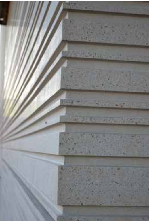
Providing a polished finish on the panels requires grinding off most of the top layer of paste to produce a shiny appearance. Photo: Gate Precast Co.
