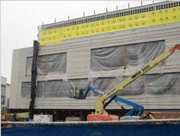
The outpatient clinic for Bridgeport Hospital being constructed in Trumbull, Conn., features architectural precast concrete panels with 4-inch fins that create an undulating pattern over the facade. Photo: Coreslab Structures (CONN) Inc.
