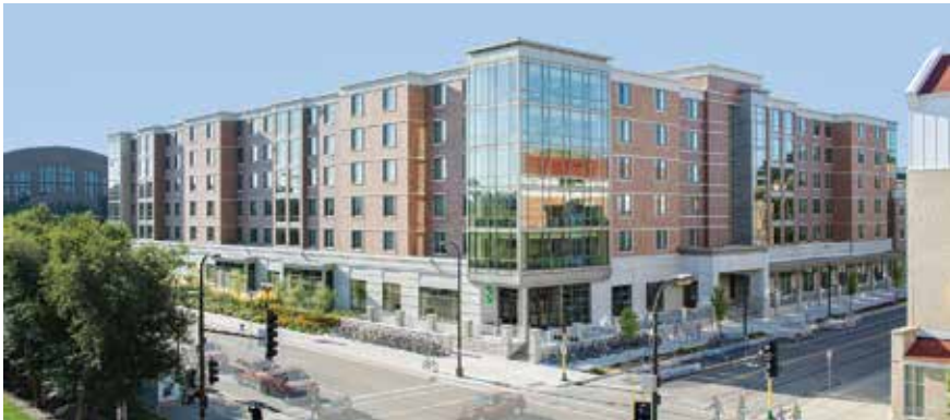
University of Minnesota 17th Avenue Residence Hall, Minneapolis MN.
