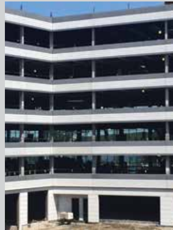
The architectural precast concrete panels cast for the 10 CityPoint office building in Waltham, Mass., features a two-color design that required special care to maintain the color segregation. Photo: Strescon Ltd.
