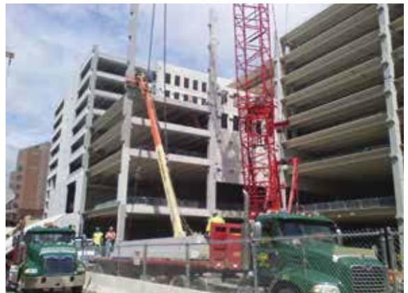
Photo: High Concrete Group LLC.
