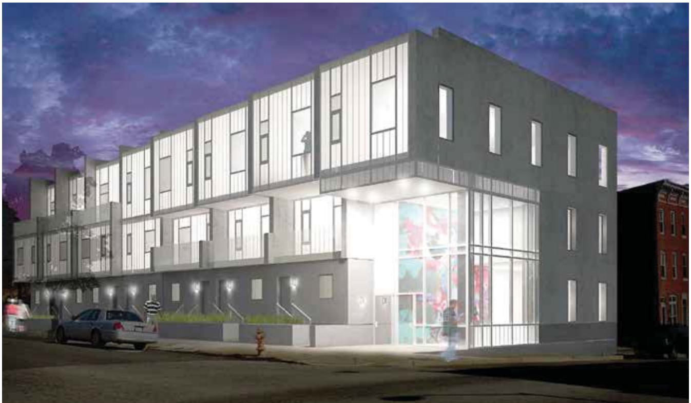
Figure 9: GRO Architects has proposed an eight-unit affordable housing project in the Oliver section of Baltimore, Md., utilizing precast concrete for the foundation, wall, and floor and roof systems. Credit: GRO Architects.
