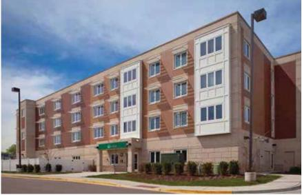
The 32,000-square-foot Myers Place residential building in Mount Prospect, Ill., combines four finishes in its load-bearing precast concrete wall panels. The facility offers affordable housing for people with mental or physical disabilities as they move towards recovery or self-sufficiency.
