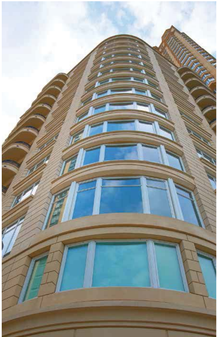
Curved precast concrete spandrels frame the large expanses of glass used at the towers' corners to create a welcoming street presence. The precasters interpreted the original architectural drawings to create details in the precast concrete panels to achieve the intended goals. Photo: High Concrete Group LLC.
