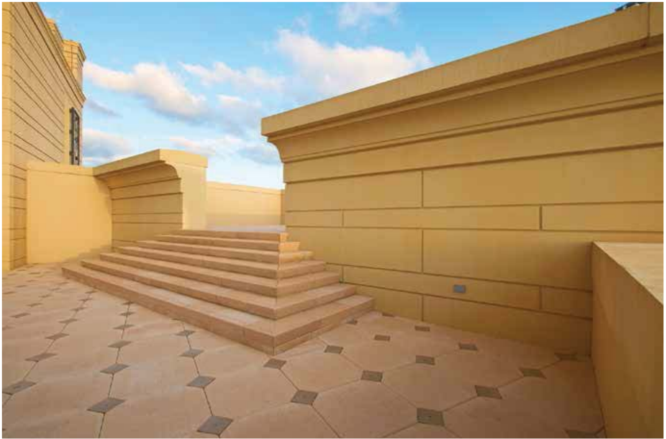
Penthouse residences feature extensive balconies with decorative architectural precast concrete components, including detailed cornices. Photo: High Concrete Group LLC.
