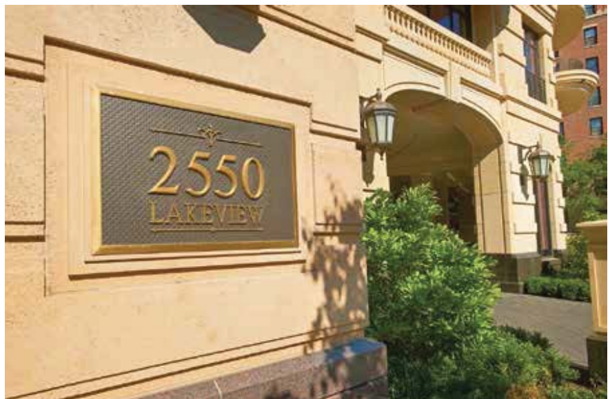
Black-granite and limestone veneer pieces were field-applied to the lower three levels of the building, providing visual interest at pedestrian level. Photo: High Concrete Group LLC.
