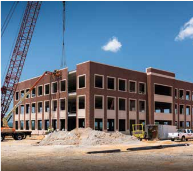
Pointe Property Group is constructing two new facilities, the 56,616-square-foot, three-story Lee Pointe speculative office building and the 17,037-square-foot, four-story Gunbarrel Suites, using total precast concrete systems.
