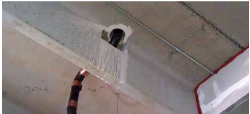
Blockouts were cast into some of the double tees to allow penetrations that plumbers could connect to an elbow, allowing plumbing to remain set in the design. Photo: FDG Inc.
