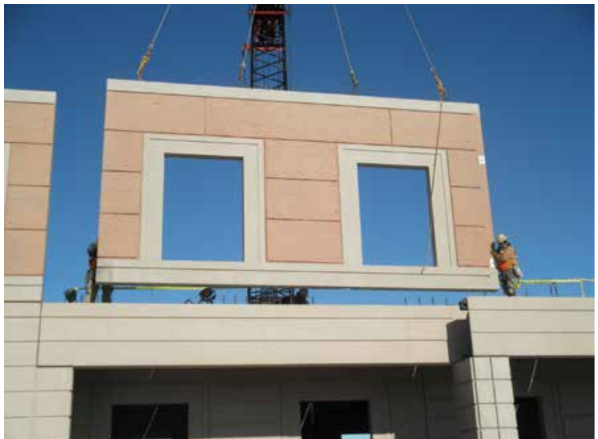
Panels feature several colors, reveals, and a variety of cutouts. Combining colors and textures into one panel reduced the piece count and sped up the erection process. Photo: FDG Inc.
