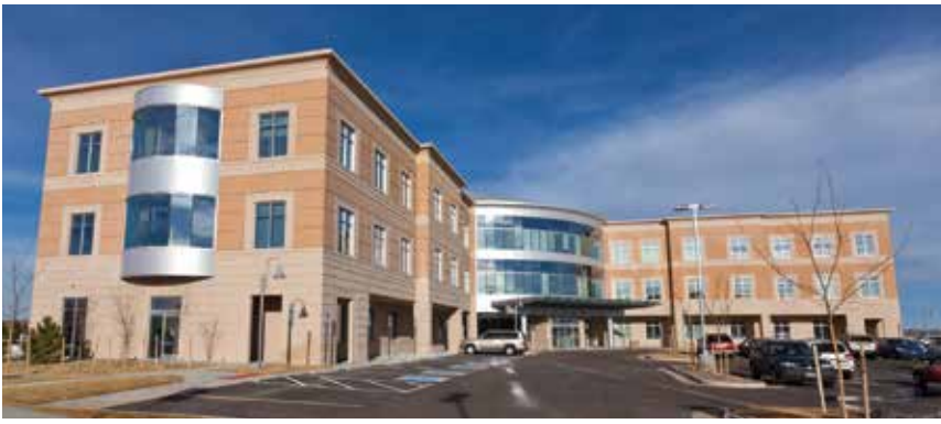
Two-story bay windows reflect the rounded curtain wall used at the entry. The windows rest on a curved precast concrete slab that cantilevers off the wall panels. Photo: Rocky Mountain Prestress.
