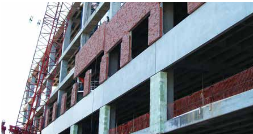
Only 24 weeks were required to erect the entire structure, including both the podium or base section and the towers. Photo: Gate Precast Co.
