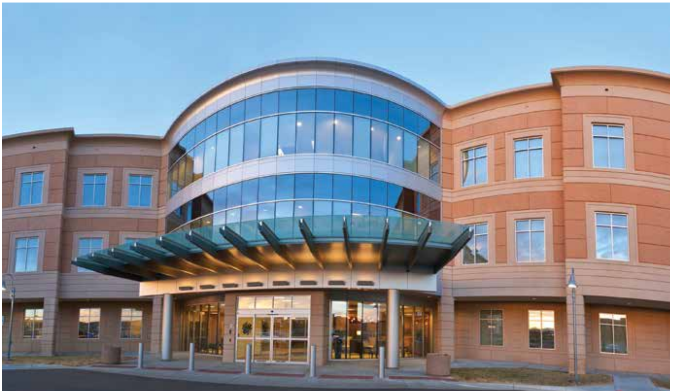
When the original steel and masonry design for The Center at Lincoln, a skilled nursing facility in Parker, Colo., proved economically unviable, a total precast concrete system was used. It consisted of 64-foot-long double tees, columns, beams, and load-bearing architectural wall panels. Photo: Rocky Mountain Prestress.
