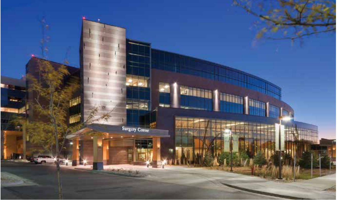
Averra Health's Prairie Center Cancer Institute in Sioux Falls, S.D., features precast concrete panels with inset thin brick, inset stone and several textures on the panels, saving more than $1 million over the original handset-brick design. Opened in 2010, the building set a new standard for the company in reducing energy consumption, using environmentally friendly construction materials, and sourcing materials locally. Gage Brothers in Sioux Falls fabricated the components. Photo: Averra Health.
