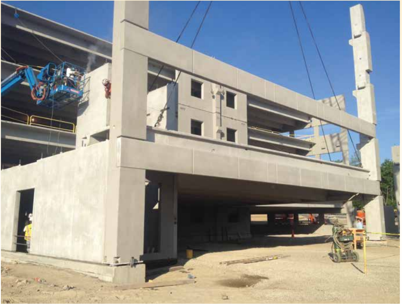
The first phases of the $500-million University Station project features 550,000 square feet of retail space and a 350-luxury residential development. The residences will wrap about a central precast concrete parking structure.
