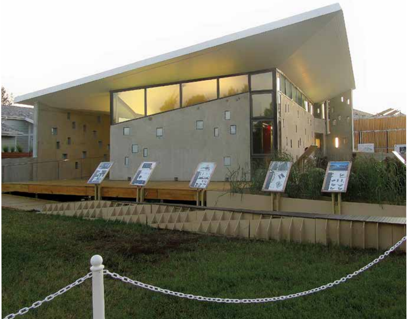
Figure 3: eNJoy! House—New Jersey Institute of Technology and Rutgers University, 2011, U.S. Department of Energy Solar Decathlon competition. Credit: Solar Team NJ.
