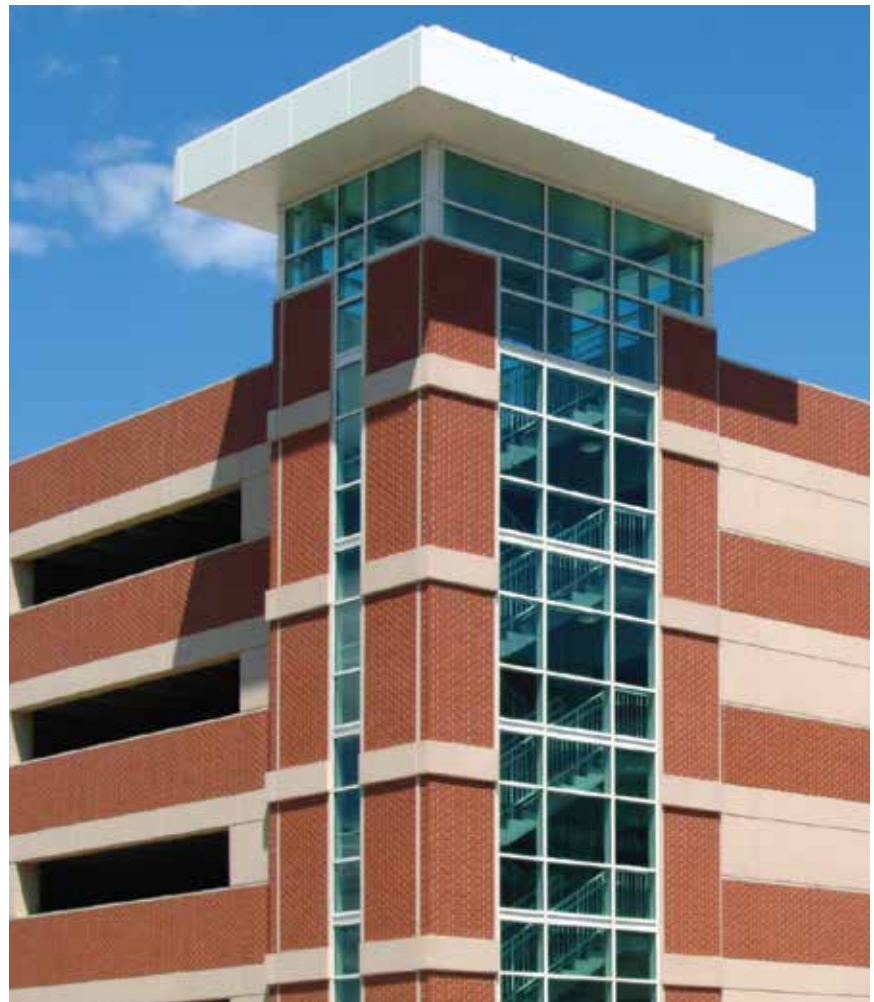
Denver Health Center's parking structure features architectural panels of combined texture palette with thin brick cast in architectural acid-washed concrete. Photo: Fred J. Fuhrmeister/Time Frame Images
