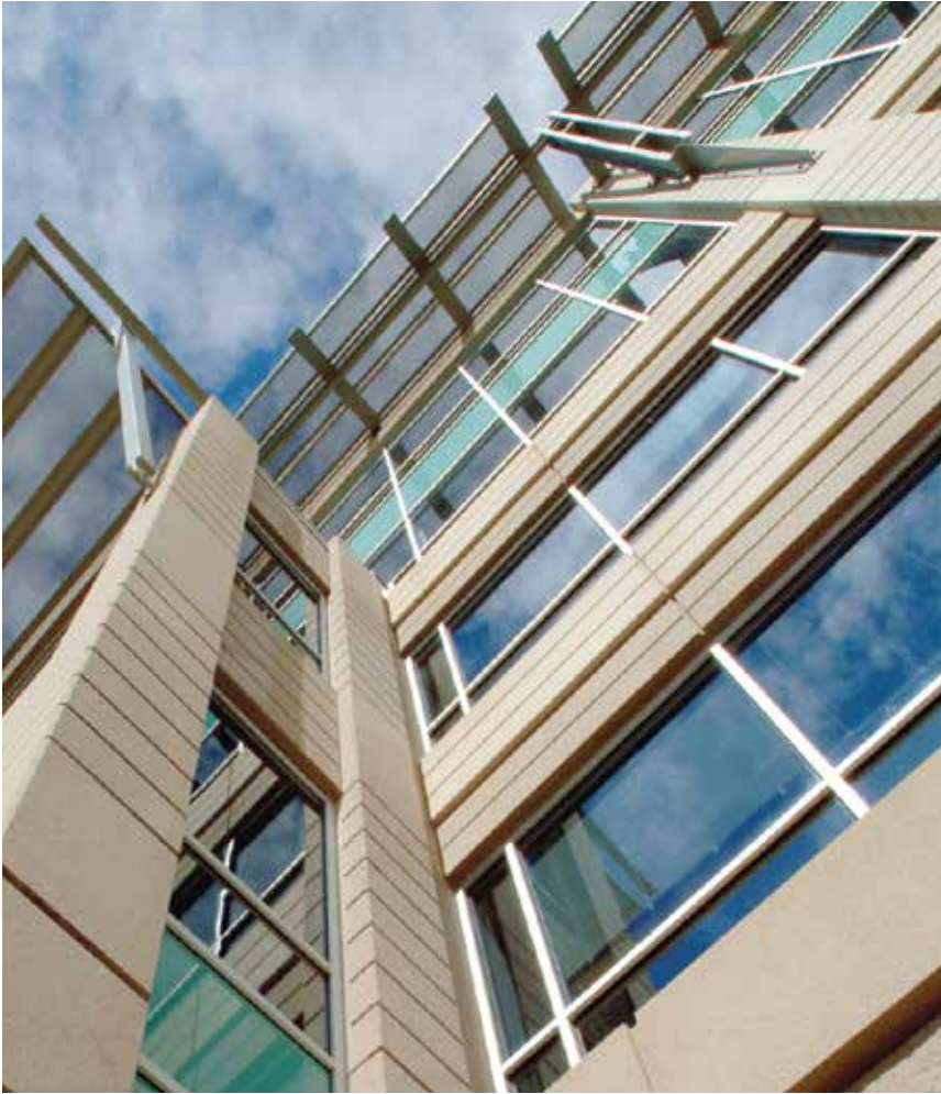
Circle Point features multi-color precast architectural panels of combined texture with deep reveals and a light acid etch finish. Photo: Fred J. Fuhrmeister/Time Frame Images
