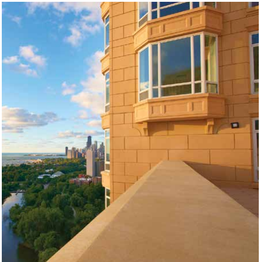
Bay windows framed with precast concrete spandrels add visual depth and enhance scenic views from every floor. Photo: High Concrete Group LLC.
