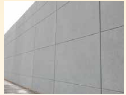
A 29,581-square-foot Kia dealership is being constructed in McDonough, Ga., using 143 9-inch-precast concrete panels with a pigment and medium sandblast finish.
