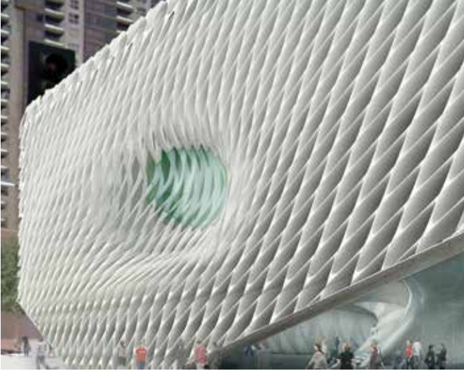
The Broad Museum in Los Angeles, Calif., received the Sidney Freedman Craftsmanship Award. Willis Construction Co. Inc. in San Juan Bautista, Calif., produced the exterior panels.
