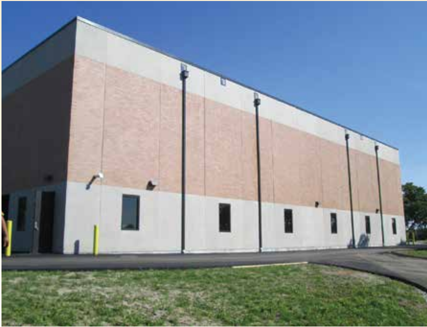
The new Water Treatment facility for the City of Newport, R.I., features precast concrete panels with a light sandblasted finish and a wide horizontal band of embedded thin bricks breaking up the mass.
