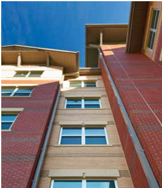
Minimizing scale and projecting a residential image were key reasons that architectural precast concrete panels with embedded thin brick were chosen to clad eight new dormitories at Newing College at Binghamton University in Vestal, N.Y. Precast concrete's speed of erection also was a key factor, as the dorms had to come on line quickly to accommodate student needs.
