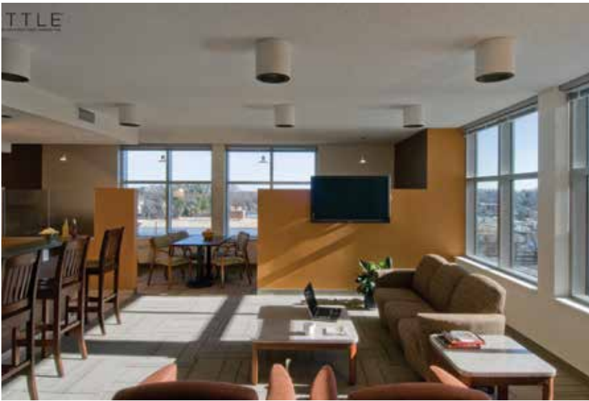
Catholic University of America, Opus Hall left the interior side of the precast envelope system exposed providing a durable, mold-resistant, interior finish. This approach also helps the structure take advantage of the thermal mass properties of precast concrete. Photo credit: Photo © John Cole 2009 / Image provided by Little
