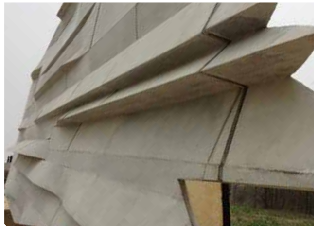
The architect, steel fabricator and precaster collaborated through building information modeling (BIM). The panels were designed with a 6 1/2 in. nominal thickness with 2 in. recesses and 8 in. projections. Photo: Gate Precast Co.
