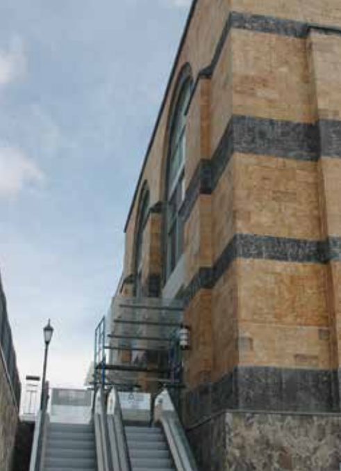
A multitude of stone appearances were created from architectural precast concrete to add a distinctive style to the massive Paseo Altozano (Altozano Walkway) shopping center in Morelia, Michoacan, Mexico. Rubber molds made from actual stones, including slate, ensured the accuracy of the precast concrete appearances. A variety of finishes added texture.
