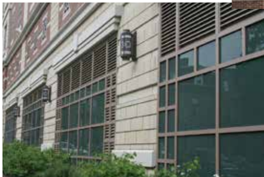
A traditional tripartite design with faux windows and elaborate details, including embedded thin brick in the architectural precast concrete panels, help the façade of the Central West Garage in Lancaster, Pa. fit in with its neighbors. The all-precast concrete structural system was connected on each level with an existing adjacent parking structure.
