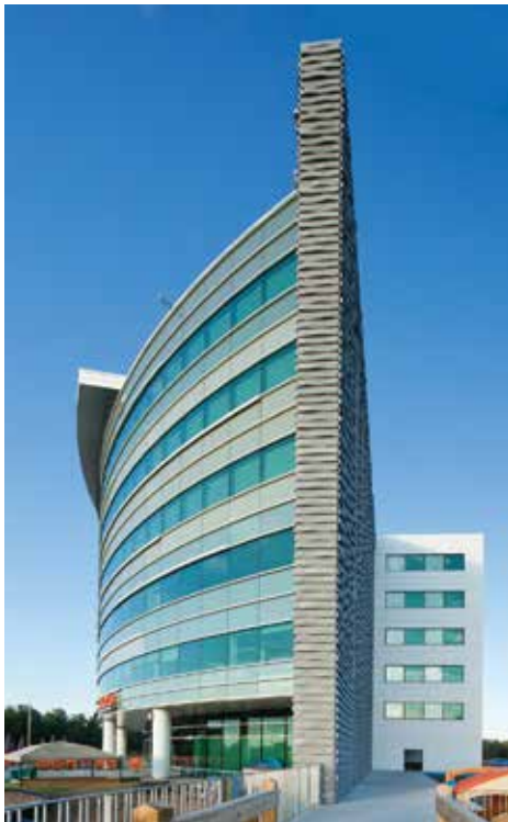
The Place de L'Escarpement commercial building in Quebec provides a bold, contemporary look that was economical and quick to construct thanks to the use of architectural precast concrete panels. Waves in the panels, designed by an artist working with the architect and precasters, were created with formliners, and a gray concrete created with black pigment.
