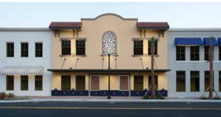
Decorative touches, ranging from brick and tile to awnings, cornices, and colorful paint, create the look of retail storefronts for a new precast concrete parking structure in downtown Winter Haven, Fla. Panels were overlapped to create a varying rhythm to the façade, and a variety of lighting fixtures minimize light overflow and mimic retail appearances. Photo courtesy of Mike Potthast, Potthast Studios
