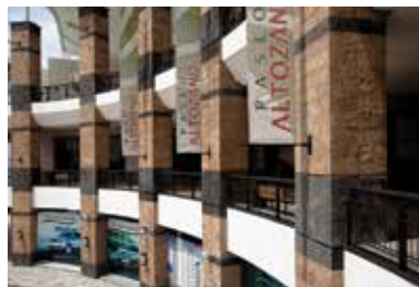
A multitude of stone appearances were created from architectural precast concrete to add a distinctive style to the massive Paseo Altozano (Altozano Walkway) shopping center in Morelia, Michoacan, Mexico. Rubber molds made from actual stones, including slate, ensured the accuracy of the precast concrete appearances. A variety of finishes added texture.
