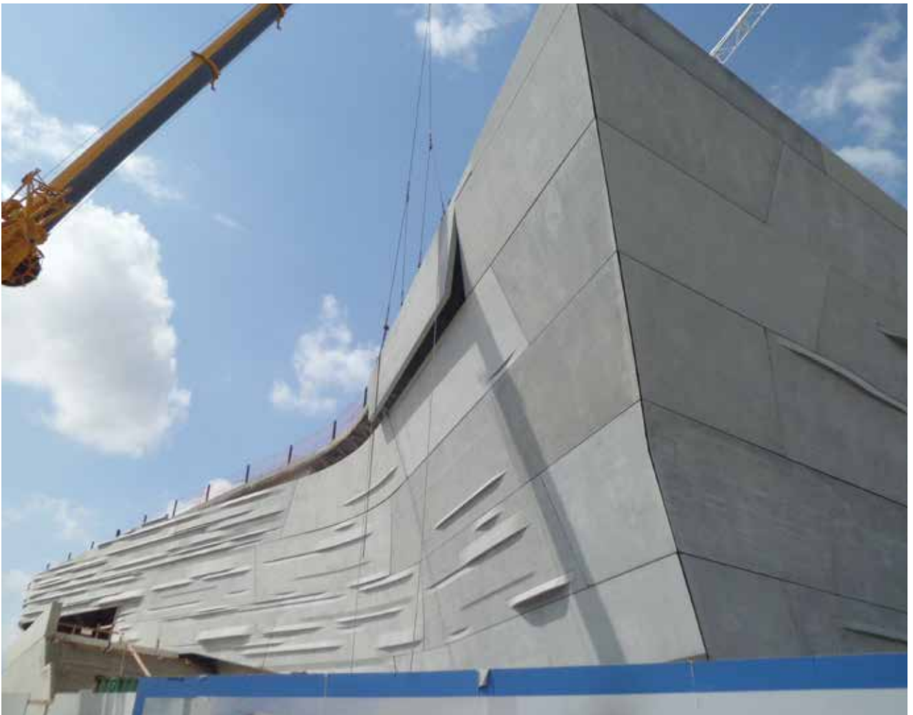
The panels were erected in a careful sequence to avoid overloading one side of the structure. Work began at the base and went around the perimeter, connecting each panel to the next and to the frame. Photo: Gate Precast Co.
