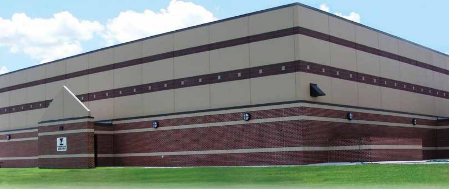
Greenwood Schools Safe Room/Gymnasium Greenwood, Arkansas
