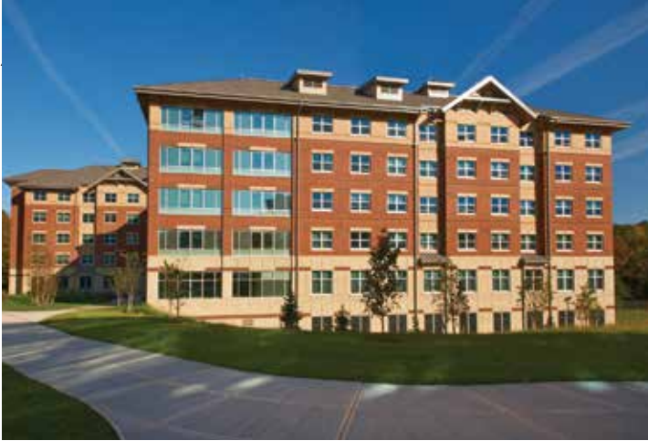
Minimizing scale and projecting a residential image were key reasons that architectural precast concrete panels with embedded thin brick were chosen to clad eight new dormitories at Newing College at Binghamton University in Vestal, N.Y. Precast concrete's speed of erection also was a key factor, as the dorms had to come on line quickly to accommodate student needs.
