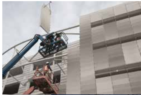
The high-profile parking structure at the UC Davis Medical Center in Sacramento features aluminum louvers and other metal decorations attached to the precast concrete spandrel panels. Each set of louvers is angled slightly differently, to cast different shadows through the day and imply movement.
