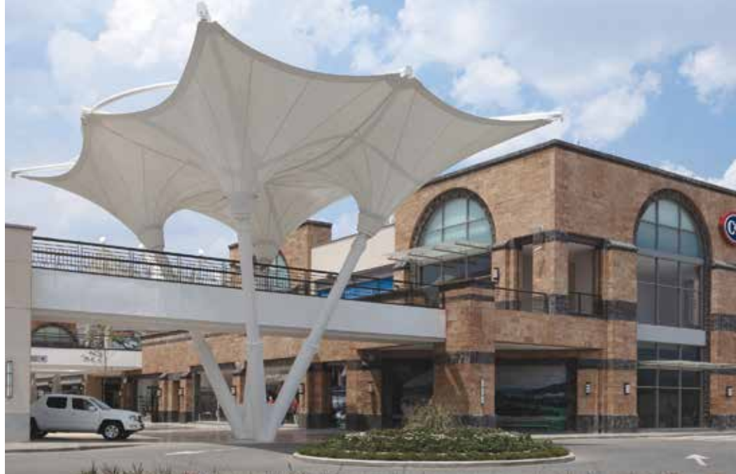
A multitude of stone appearances were created from architectural precast concrete to add a distinctive style to the massive Paseo Altozano (Altozano Walkway) shopping center in Morelia, Michoacan, Mexico. Rubber molds made from actual stones, including slate, ensured the accuracy of the precast concrete appearances. A variety of finishes added texture.
