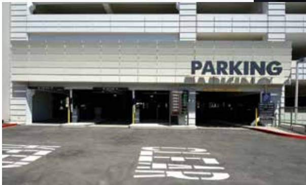
The high-profile parking structure at the UC Davis Medical Center in Sacramento features aluminum louvers and other metal decorations attached to the precast concrete spandrel panels. Each set of louvers is angled slightly differently, to cast different shadows through the day and imply movement.
