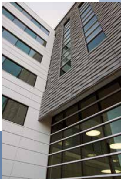
The Place de L'Escarpement commercial building in Quebec provides a bold, contemporary look that was economical and quick to construct thanks to the use of architectural precast concrete panels. Waves in the panels, designed by an artist working with the architect and precasters, were created with formliners, and a gray concrete created with black pigment.
