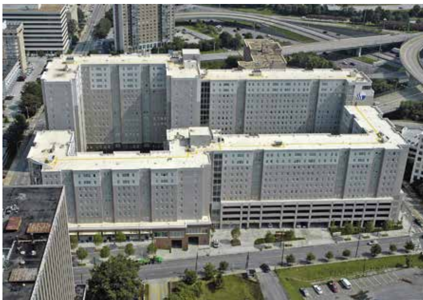
The four buildings making up the complex were designed to create a large courtyard at their center to help pull daylight into all of the housing units, brightening the spaces and saving on lighting costs.
