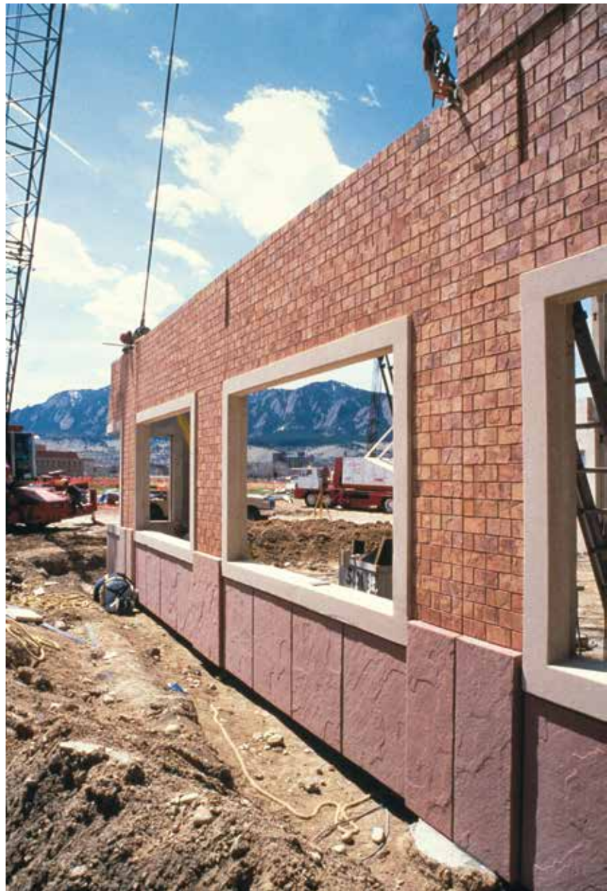
This precast concrete panel combines three finishes into one efficient element saving time, material and money.
