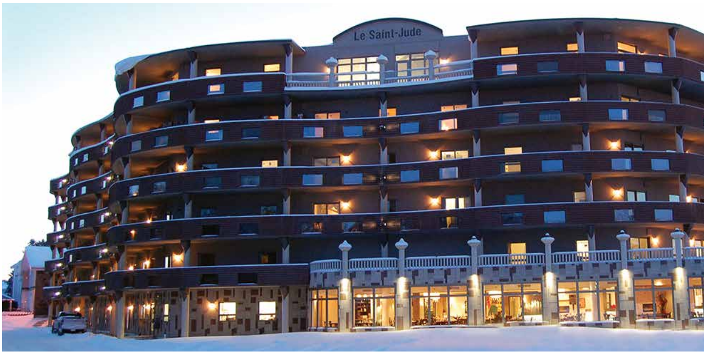
The six-story Residence Le Saint-Jude retirement residence in Quebec in Alma, Quebec, features a striking exterior comprising architectural precast concrete panels in three finishes and multiple curving shapes. Its total-precast concrete structural system was designed to provide strong seismic and wind-force protection and features precast concrete beams, columns, slabs, balconies, and stairs. Photos courtesy of BPD.
