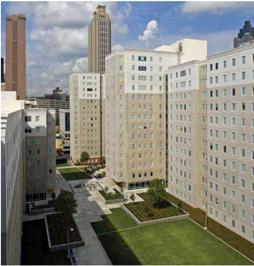
Three finishes were used on the precast concrete panels, comprising a white sandblast finish across the top of the majority of the buildings; a buff sandblasted finish below that on the bulk of the buildings; and inset thin bricks, used at pedestrian level.
