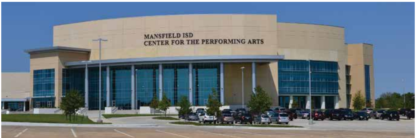
The Center for Performing Arts in Mansfield, Texas, features thermally efficient, pre-insulated precast concrete panels that cut energy costs while providing a maintenance-free exterior envelope. Photos courtesy of Gate Precast Co.
