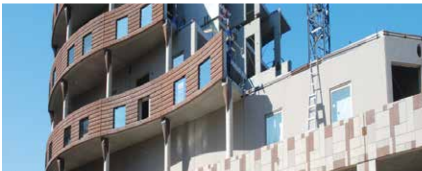
The six-story Residence Le Saint-Jude retirement residence in Quebec in Alma, Quebec, features a striking exterior comprising architectural precast concrete panels in three finishes and multiple curving shapes. Its total-precast concrete structural system was designed to provide strong seismic and wind-force protection and features precast concrete beams, columns, slabs, balconies, and stairs. Photos courtesy of BPD.
