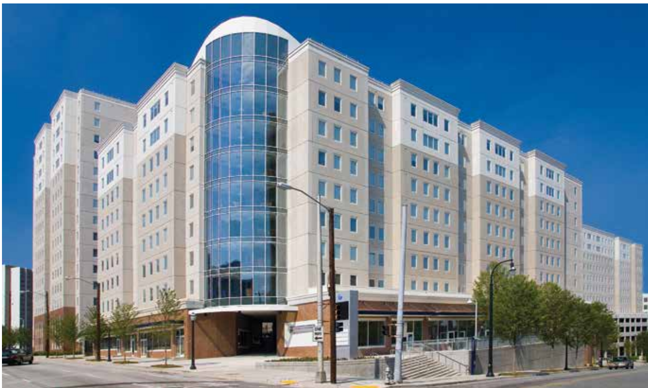
Georgia State's University Commons 2000-bed residential hall features insulated precast concrete wall panels that provided a strong, permanent appearance, allowed the building to be completed earlier than scheduled, saved $1 million in construction costs and maximized energy savings over the building's life. All photos courtesy of Metromont Corp..
