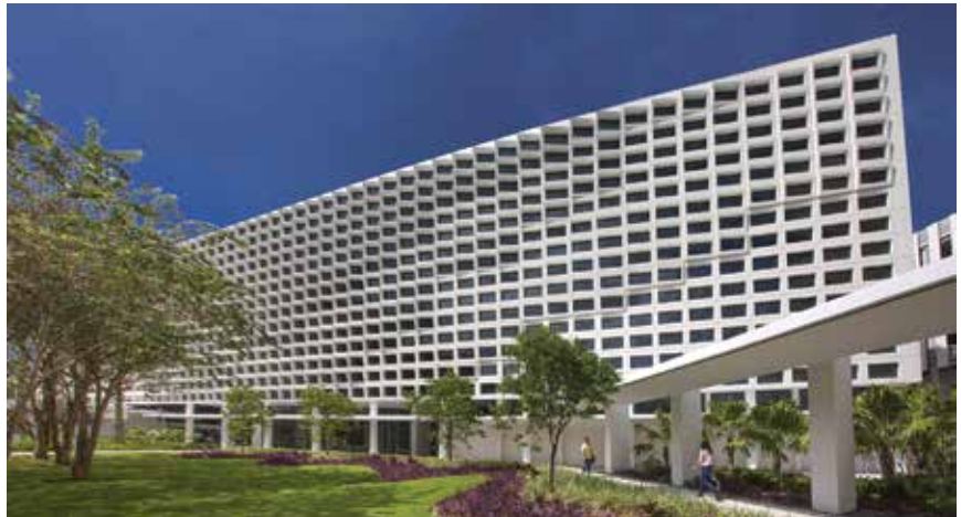
FIU Science Classroom Complex features precast sunshading elements. Photo: Miami in Focus.
