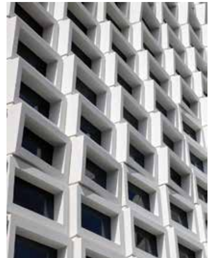
Actual photo of precast window openings that tilt in multiple directions.
