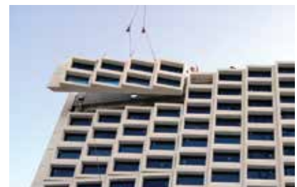
Topping out enclosure with last window panel. Photo: DPR Construction.
