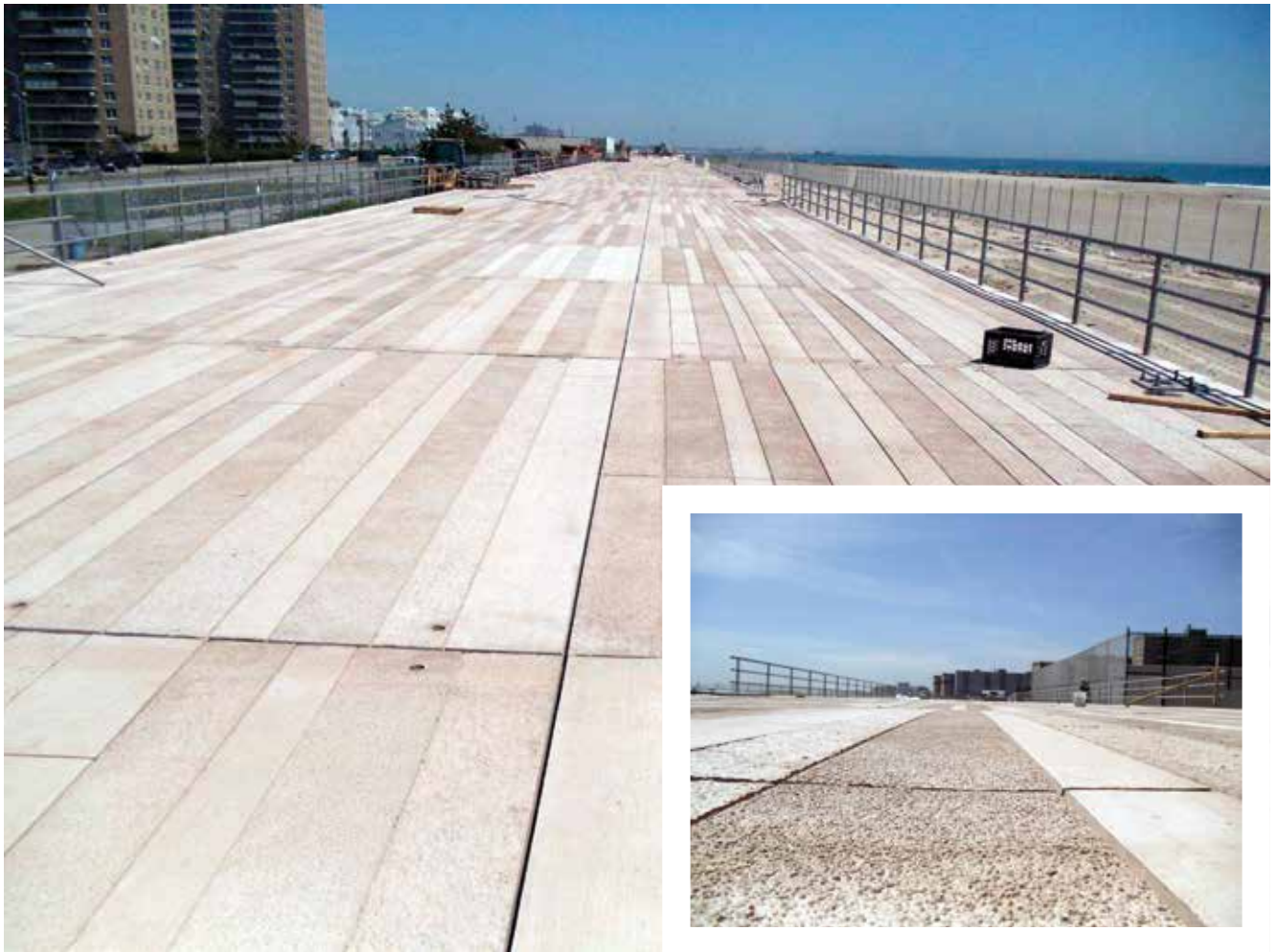
Precast concrete panels, formed to resemble five textured planks, were used in rows of five to produce an upgraded 10,000-linear-foot boardwalk in Queens, N.Y. The panels withstood Hurricane Sandy, the only portion of the boardwalk to remain intact. Photos: Steve Kenep, U.S. Concrete Precast Group.
