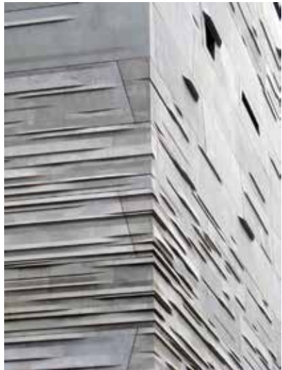
Precast panels were digitally modeled in the design assist process which allowed greater integration/coordination with other building materials. All photos: Gate Precast.
