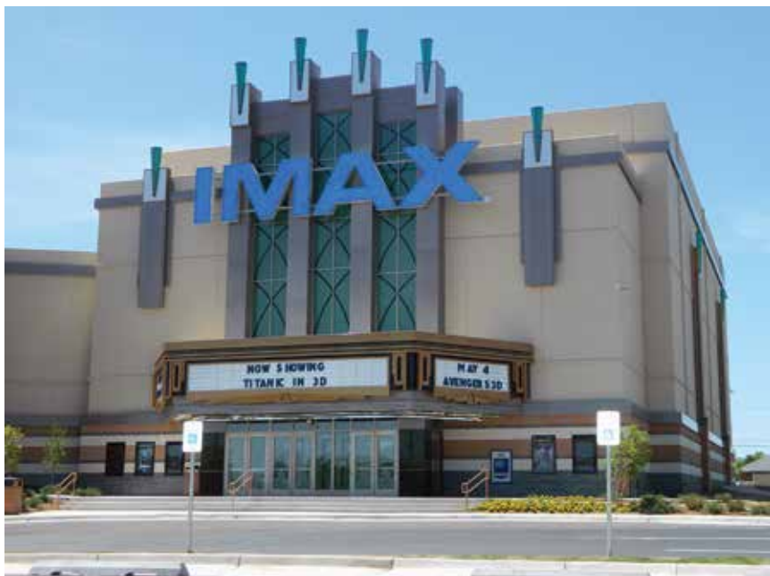
A number of factors allowed the precast concrete panels on the Imax Theater addition to the Warren Theater in Moore, Okla., to survive intact when tornadoes hit the area in May. Patrons survived without injury, and the theater was turned into an emergency center. Photos: Coreslab Structures (OKLA), Inc.
