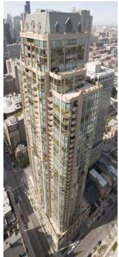
The Pinnacle residential tower in Chicago features architectural precast concrete panels in two finishes to complement the French limestone at the base and blend the building with the nearby Cathedral District.
