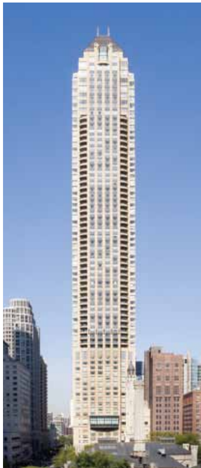
Park Tower in Chicago, which combined hotel, condominium and retail functions, was the first high-profile project for Lagrange. The building is one of the tallest in the world to be clad with architectural precast concrete panels, containing 3,152 pieces.
