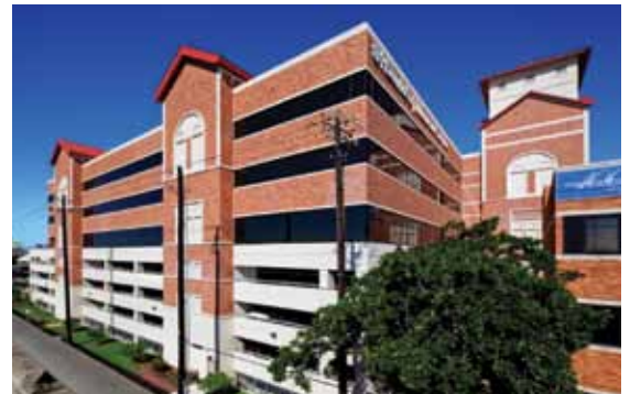
The Medical Midtown Office Building on the St. David's Medical Center campus in Austin, Texas, features doctors' offices and parking designed with a total-precast concrete structural solution. Precast was used to minimize maintenance and allow for rapid shell construction, which was accomplished despite the tight site.
