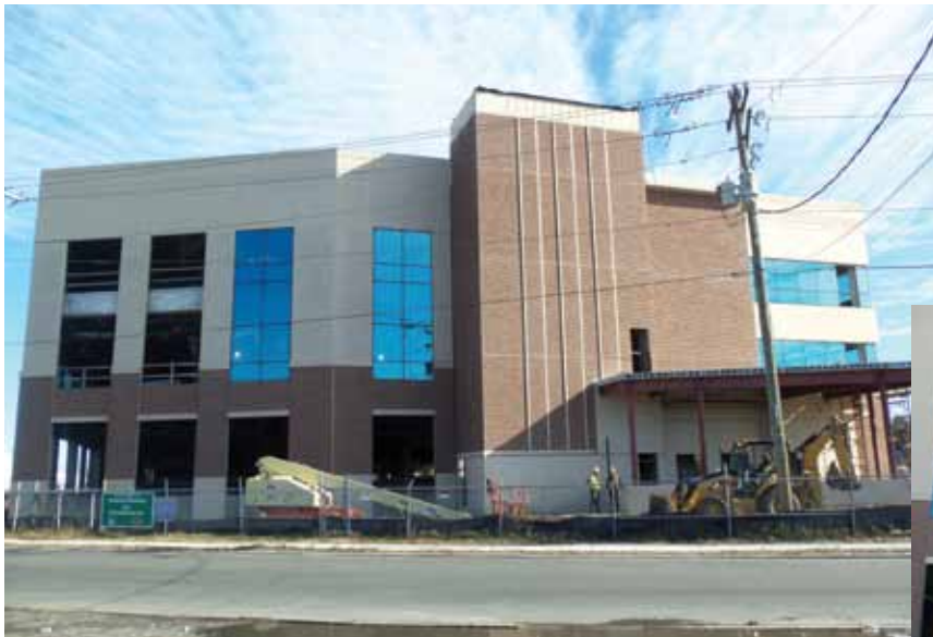
The Bus Maintenance facility for the Hampton Roads Transit company in Norfolk, Virginia, consists of office, bus-maintenance facilities, refueling and washing space, and office space. The office and parking facilities feature total-precast concrete structural solutions, while the others feature architectural precast concrete panels, most of which include embedded thin brick to provide a masonry façade appearance.
