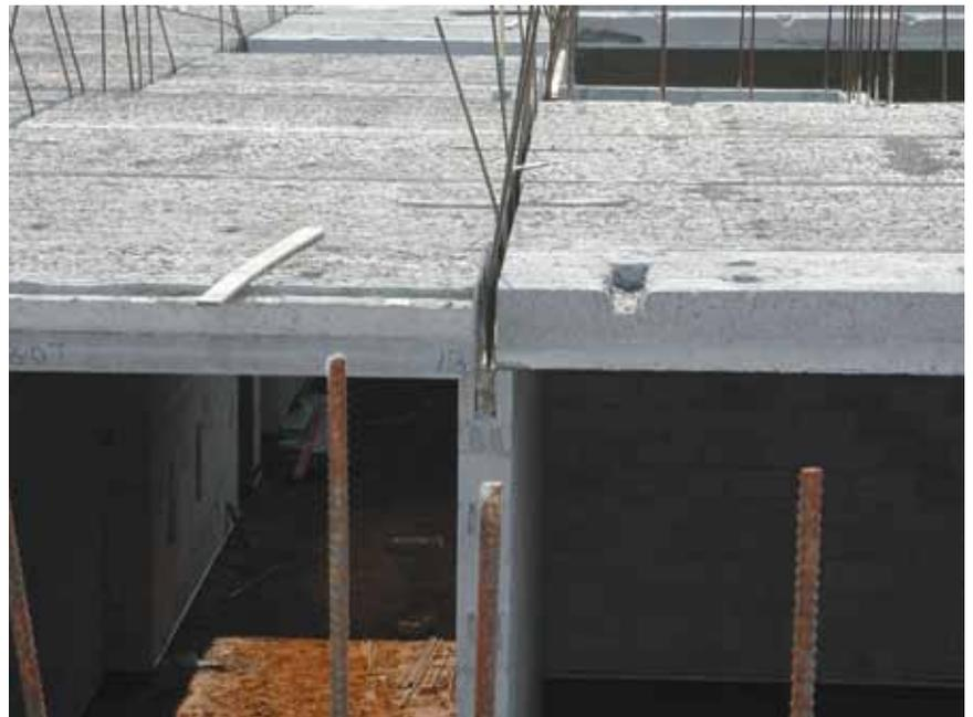
*Precast concrete floor plank often interfaces with reinforced concrete masonry bearing walls, creating a mix of materials that must be addressed, either in design or in the field.*
