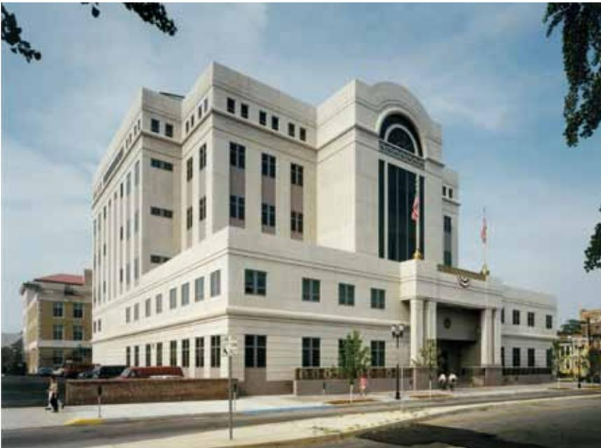
*Precast wall panels provided a one-component barrier-wall or face-sealed design solution at the Mitchell H. Cohen Court House in Camden, N.J.*
