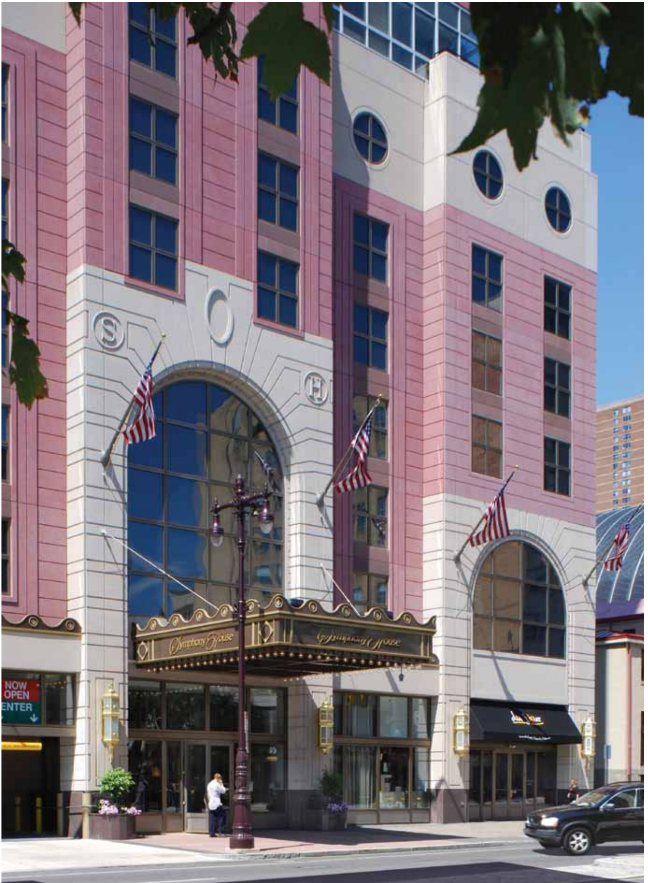
The 32-story Symphony House condominium tower in Philadelphia combines carbon-fiber reinforced architectural precast concrete panels with “punched” windows to leverage the use of daylight while providing sunlight control and high energy efficiency. BLT Architects served as the architect and interior designer. Photos: Michael Ytterberg.
