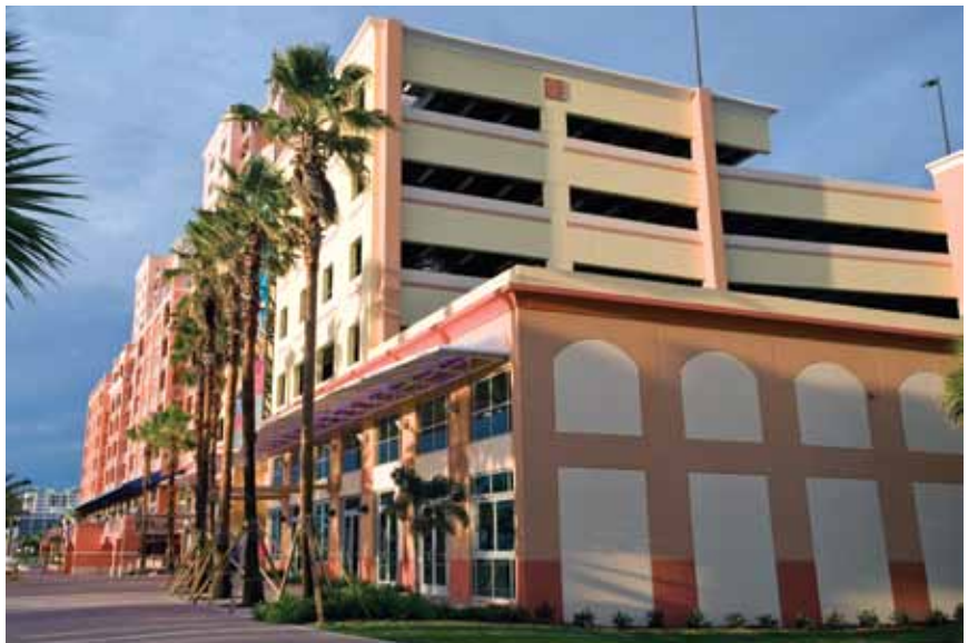
A speed ramp provides quick access to the first level of parking. It was placed above the first-floor restaurant space.
