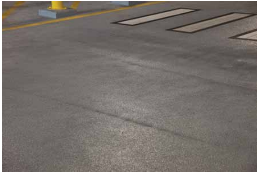
A Neoguard brand waterproofing was applied directly to the precast concrete double tees above the retail space to ensure a leak-free retail area below. Connections were cast for access from below as well to provide additional protection.
