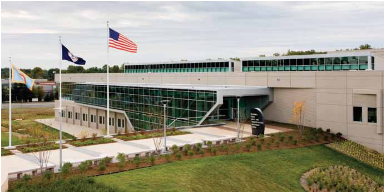
Kessler's work with HOK's Justice Group includes the recently completed McConnell Public Safety & Transportation Operations Center in Fairfax County, Va. The facility brings together several agencies to enhance the effectiveness of public-safety response, improve traffic-congestion management and respond and recover faster from major emergencies. The building features precast concrete architectural panels on its exterior, providing a dramatic look and resilience to natural and man-made disasters. Photos: Lee B Ewing.
