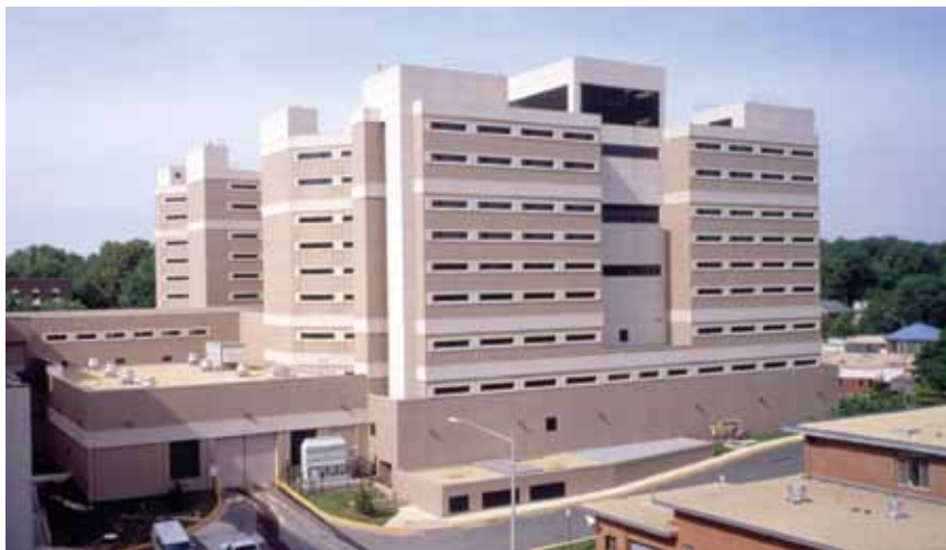
The Fairfax County Adult Detention Center expansion in Fairfax, Va., designed by Jim Kessler in 1990, was his first project to feature precast concrete. It stacked eight levels of precast concrete cells in two-unit modules on a two-story cast-in-place foundation. The building was erected quickly with modules erected as soon as they arrived at the site. Photos: Copyright Lee B Ewing.
