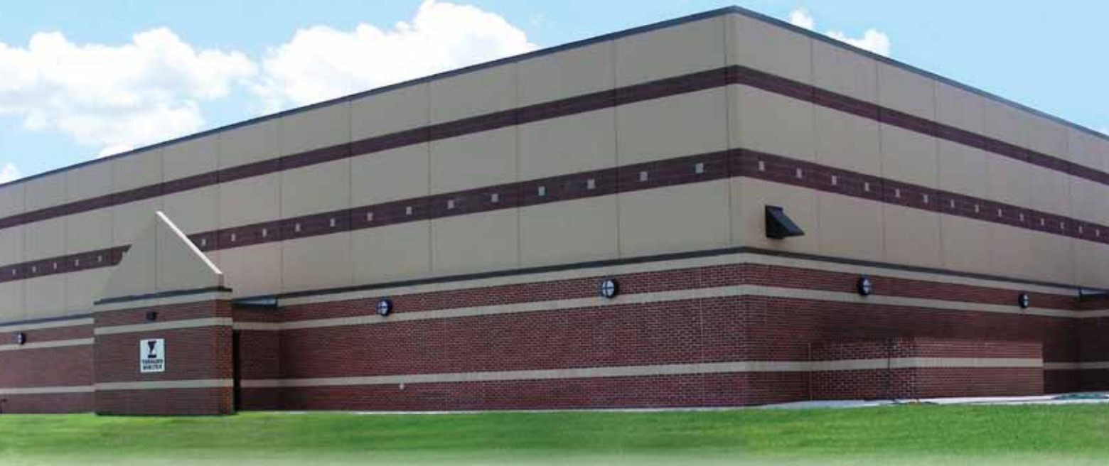
Greenwood Schools Safe Room/Gymnasium Greenwood, Arkansas
