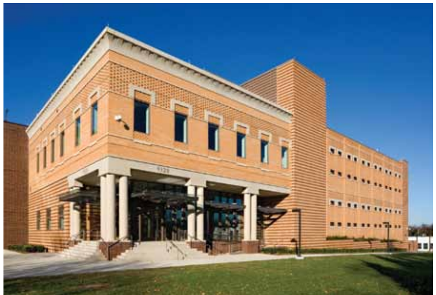
The Prince William County Adult Detention Center in Virginia features a total precast concrete structural solution, including beams, columns, double tees and double-cell units. The building contains 92 cells and features laid-up brick on precast concrete panels on its exterior to blend with the neighboring buildings. Photo: Copyright Lee B Ewing.
