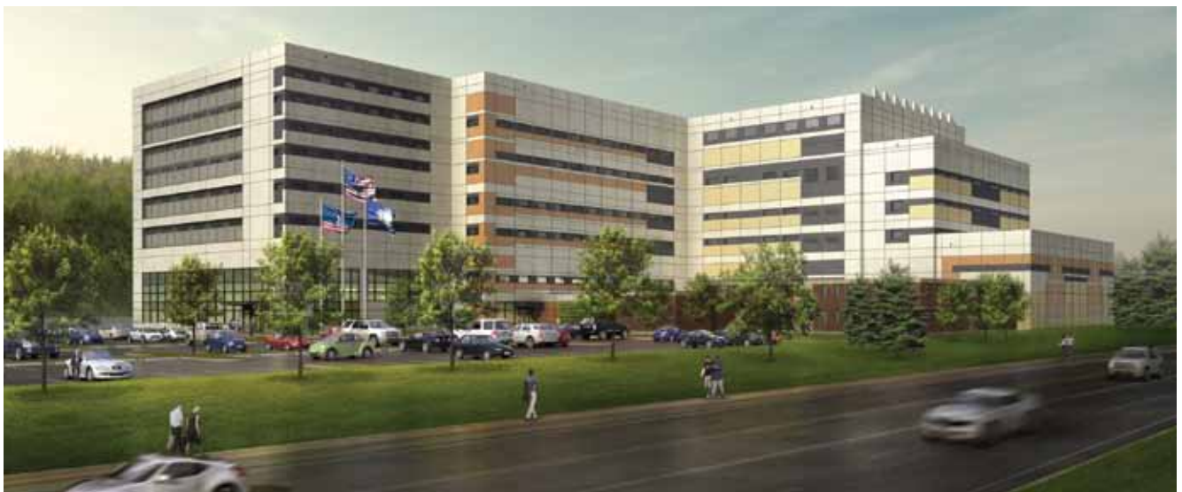
A total-precast concrete structural solution was selected for the $134.6-million, 1,032-bed Richmond Justice Center, which is now being constructed. It features quad cell units, double tees, columns, beams and exterior load-bearing architectural insulated sandwich wall panels. The panels are being cast with the use of form liners that hold thin brick which are embedded in the building façade to create a contextual and rhythmic design.
