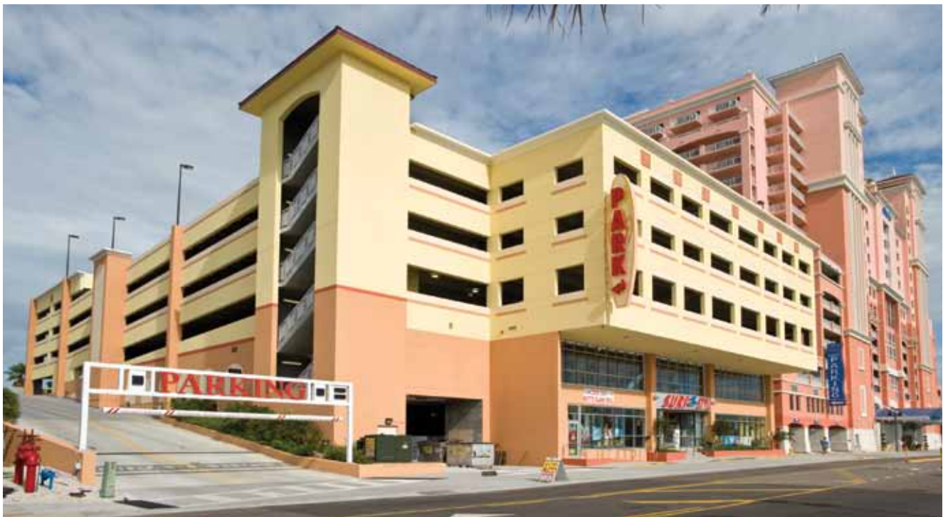
The Surf Style retail store and parking structure built along the beach in Clearwater, Fla., features a total-precast concrete structural solution that resolved a number of key challenges for the project while providing a strong aesthetic and fast erection.
