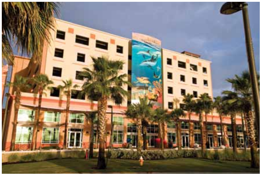
The facility includes retail and a restaurant on the first floor, with parking above. Note the artwork, a requirement by the city, which fronts a setback that was also required by the city's Beach By Design guidelines.
