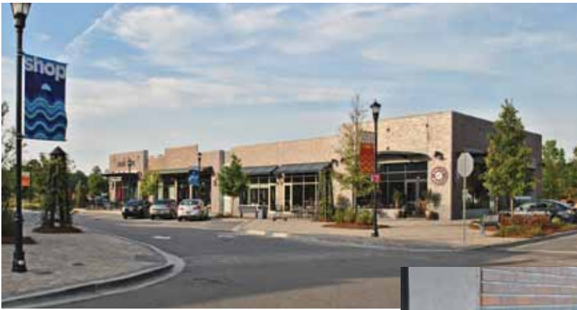
A total-precast concrete structural solution of double tees and load-bearing architectural panels provided the building shell for these two retail buildings across the street from each other in Mount Pleasant, S.C.
