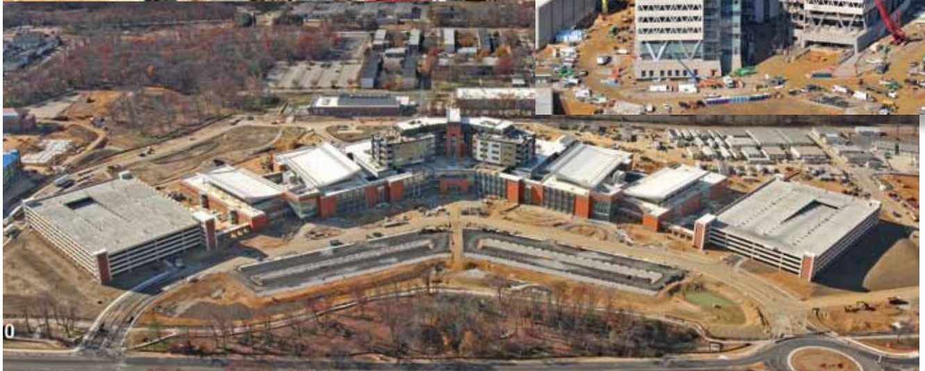
As a Base Realignment & Closure (BRAC) project, the National Geospatial Agency complex was on a fast track. To speed construction, precast concrete panels complete with wall assemblies were used to enclose the buildings. The design created distinctive architecture while meeting AT/FP requirements.
