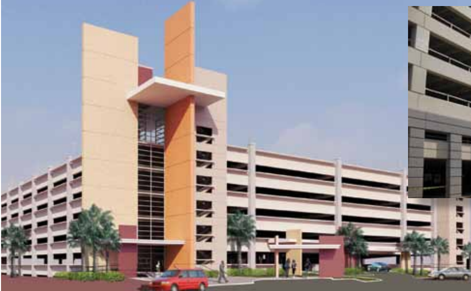
This rendering of the new precast concrete parking structure at the James A. Haley Veterans Administration facility in Tampa, Fla., shows tall vertical elements that will help visitors locate the parking facility upon arrival. Horizontal elements will shade the entries and carry through as design elements in the rest of the construction project.
