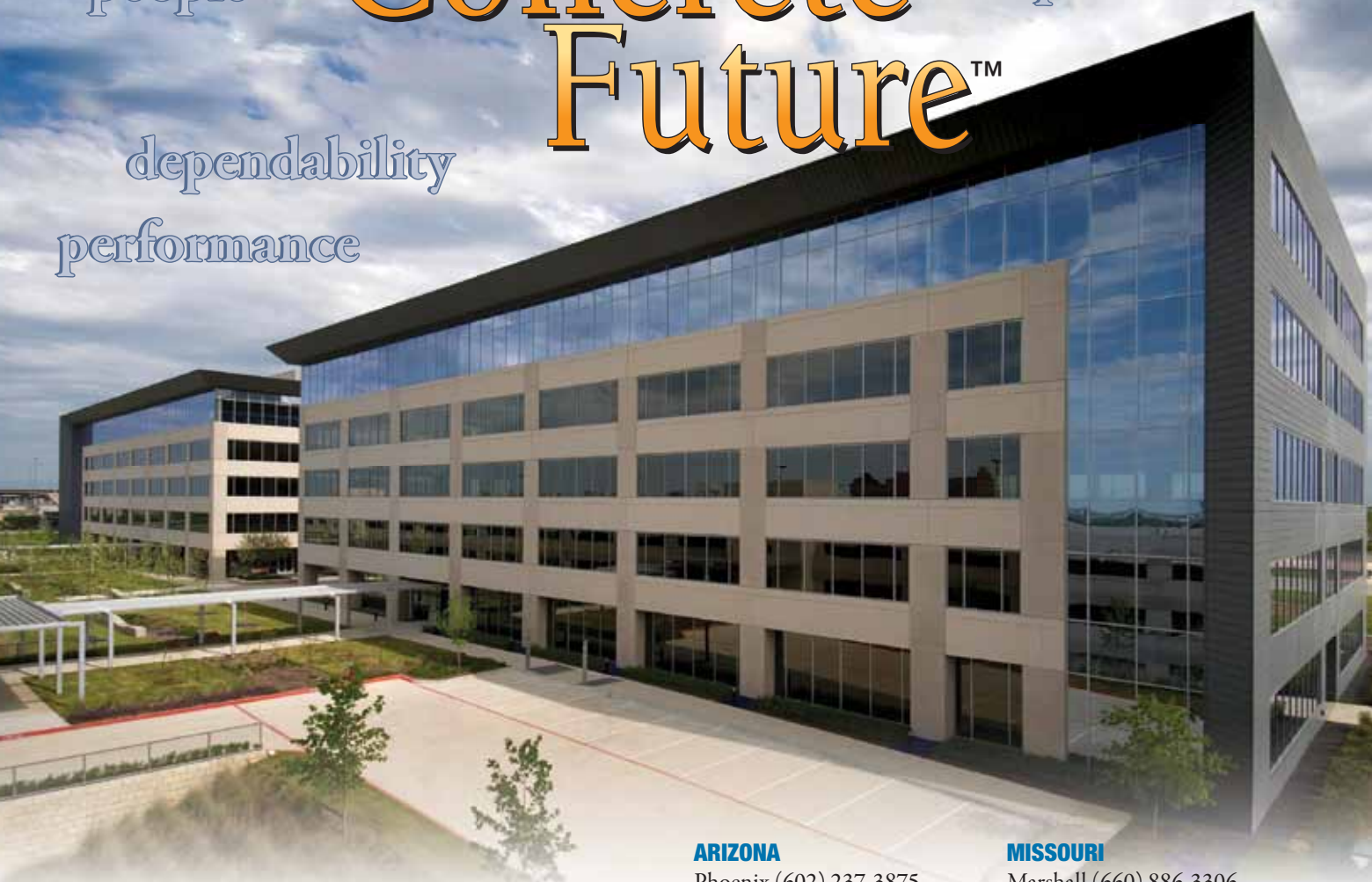
Fonterra Vista Office Buildings, Round Rock, Texas
