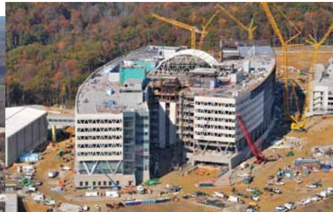
The new National Geospatial Agency campus being built on the former Engineer Proving Grounds at Fort Belvoir, Va., consists of two 1,100-foot-long, eight-story buildings connected by a six-story atrium. Built by the joint venture of Clarke/Balfour-Beatty, the project includes a large central utility plant, a parking structure, and a technical/data center.
