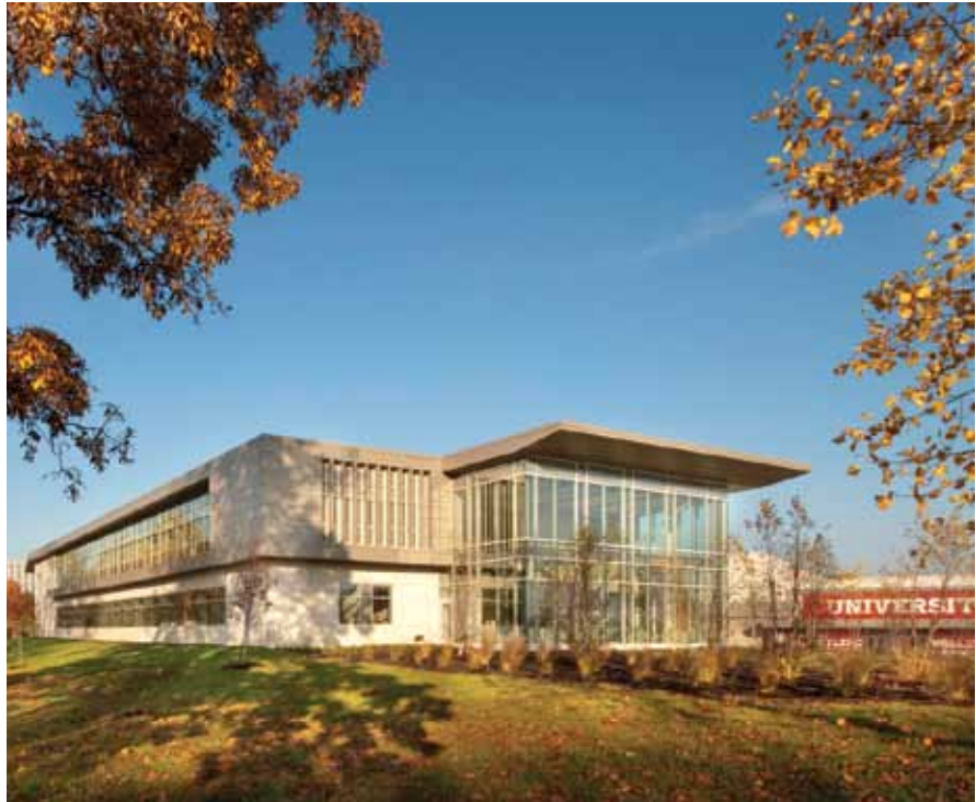
Photo courtesy of High Concrete Group LLC
