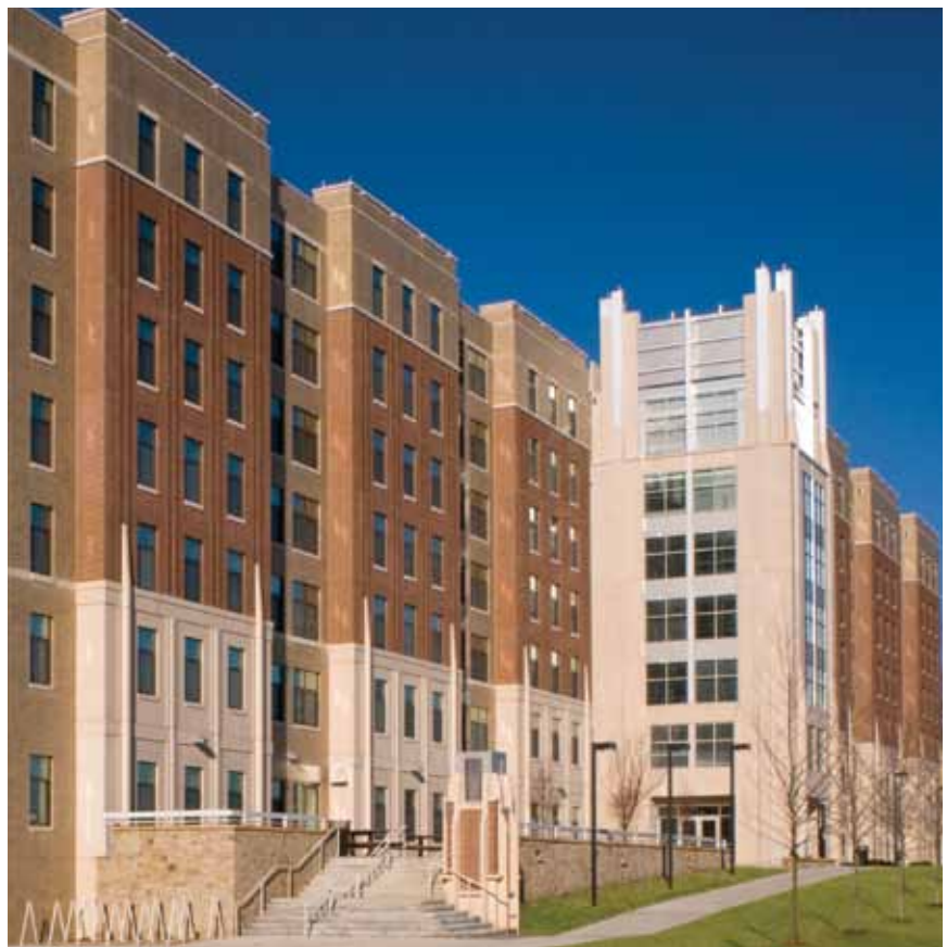
Illustration 8. The Opus Residence Hall at Catholic University of America used precast concrete insulated sandwich wall panels with embedded thin brick to create a look that blended with nearby campus buildings and also provided a highly efficient insulating wall system. Photo: Little Diversified Architectural Consulting
