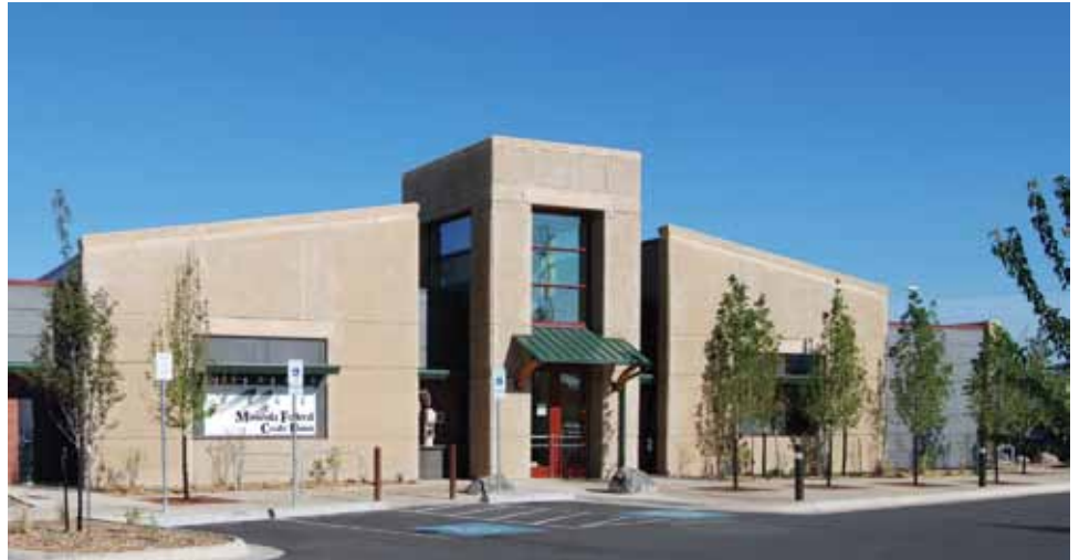
Photo courtesy of Luke Jackson, MMW Architects
