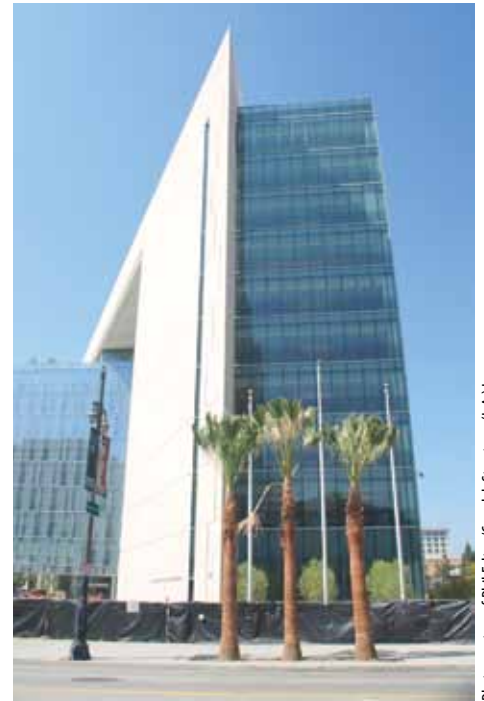
Photo courtesy of Phil Felten/Coreslab Structures (L.A.) Inc.
