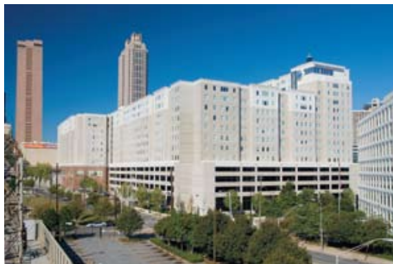
Inset brick was embedded in panels used at street-level height at University Commons, to provide the same look as other buildings in the neighborhood. Higher on the building, the panels feature a buff sandblast finish.
