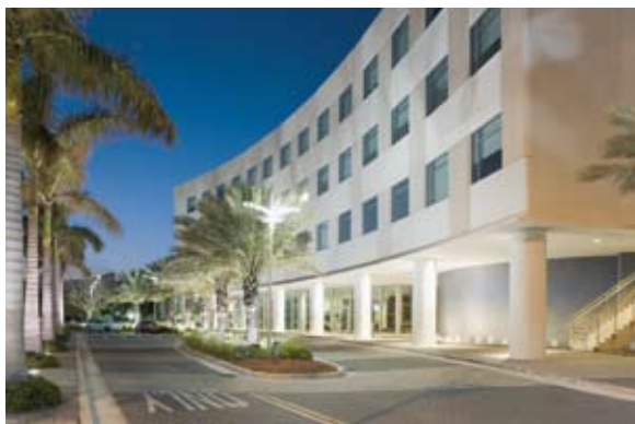
A basket-weave design was created for Sunny Isles Beach Government Center in Florida using a ribbed pattern on architectural precast concrete panels.
