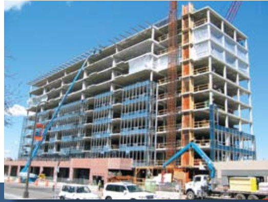
The Cobalt Condominium project in Minneapolis, Minn., features an innovative precast concrete truss system that creates column-free space on every other floor.
