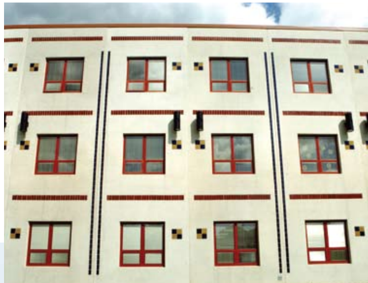
Cast-in red tile on the classroom wing of the Academy of World Languages emphasizes the precast concrete panels' horizontal lines. Photo courtesy of McGill Smith Punshon.
