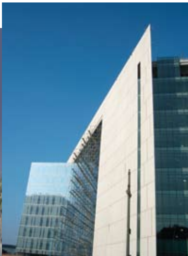
The LAPD Administration Building in Los Angeles features textured architectural precast concrete wall panels, including a west facade with tall, seemingly randomly placed windows that were in fact created with only six different wall panel forms.
