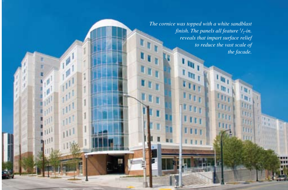
The sheer size of the University Commons project at Georgia State University magnified any design decisions, resulting in the project team selecting non-load-bearing precast concrete sandwich wall panels with 4 in. of expanded polystyrene insulation.
