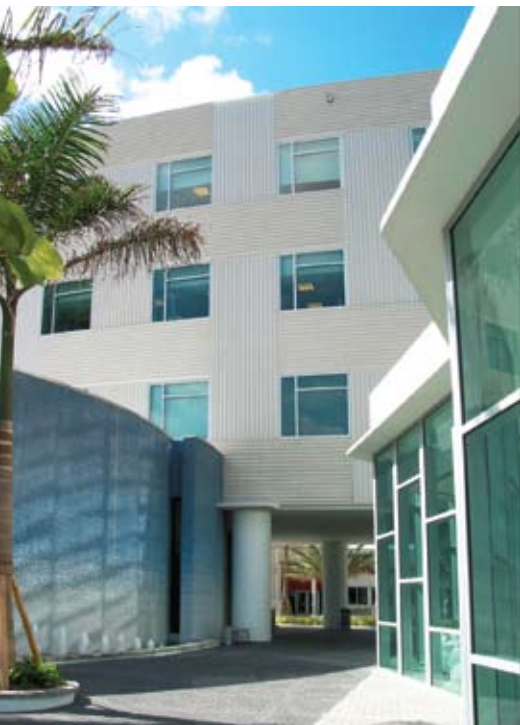
A basket-weave design was created for Sunny Isles Beach Government Center in Florida using a ribbed pattern on architectural precast concrete panels.
