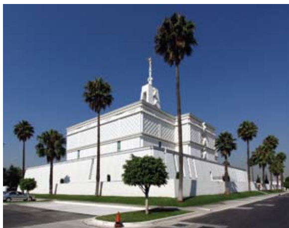
Photo courtesy of PRETECSA Archive.
