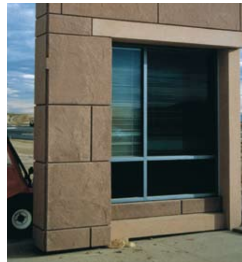
Figure 7 Mockups usually show the different shapes and finishes on typical panels.
