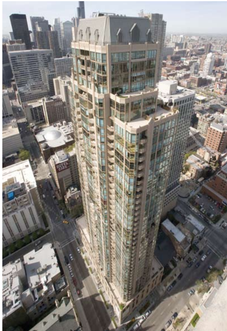
The Pinnacle residential tower in Chicago, Ill., features architectural precast concrete panels in two finishes to complement the French limestone at the base and blend the building with the nearby Cathedral District.
