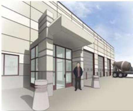
High Concrete's new maintenance building, which was designed to qualify for a Silver LEED rating, features the company's precast concrete architectural panels for its cladding.
