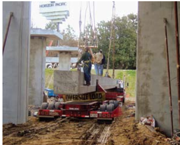
Construction workers prepare to hoist the top flange of one of Howell Mill’s beams into place.
