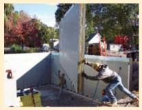
Double-wall precast system provides energyefficiency from the footings up. Photo: Dukane Precast Inc.
