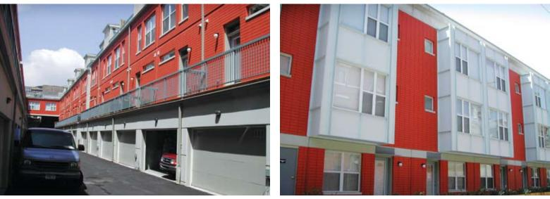
Arcadia Place in Chicago, designed by Landon/Bone/Baker Architects and developed by Dubin Residential, features stacked-bond patterned precast concrete wall panels, smooth panels with reveals, garage headers and precast concrete parapets provided by Prestress Engineering Corp. in Prairie Grove, Ill.
