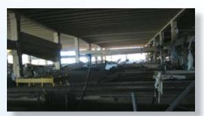
Much of the damage done to precast concrete parking structures along the Gulf Coast by Hurricane Katrina was caused by the high storm surge, which flooded the structures and caused double tees to be pushed off their supports. Otherwise, the material performed well.
