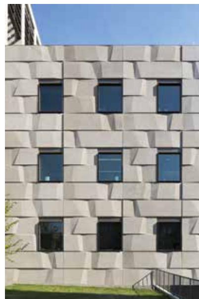
The stone texture on the courthouse's base was created by using 12 formliners combined in different ways, including flipping them 180 degrees, to create larger panels. The panels were erected in a particular sequence to avoid repetition. Each liner had a different skew, creating as much as 4 inches of offset between any two panels.
