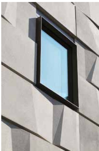
The stone texture on the courthouse's base was created by using 12 formliners combined in different ways, including flipping them 180 degrees, to create larger panels. The panels were erected in a particular sequence to avoid repetition. Each liner had a different skew, creating as much as 4 inches of offset between any two panels.
