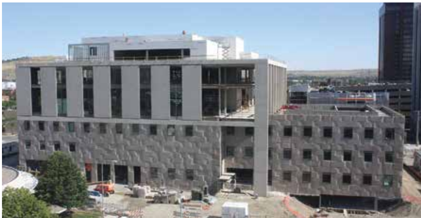
The stone texture on the courthouse's base was created by using 12 formliners combined in different ways, including flipping them 180 degrees, to create larger panels. The panels were erected in a particular sequence to avoid repetition. Each liner had a different skew, creating as much as 4 inches of offset between any two panels.
