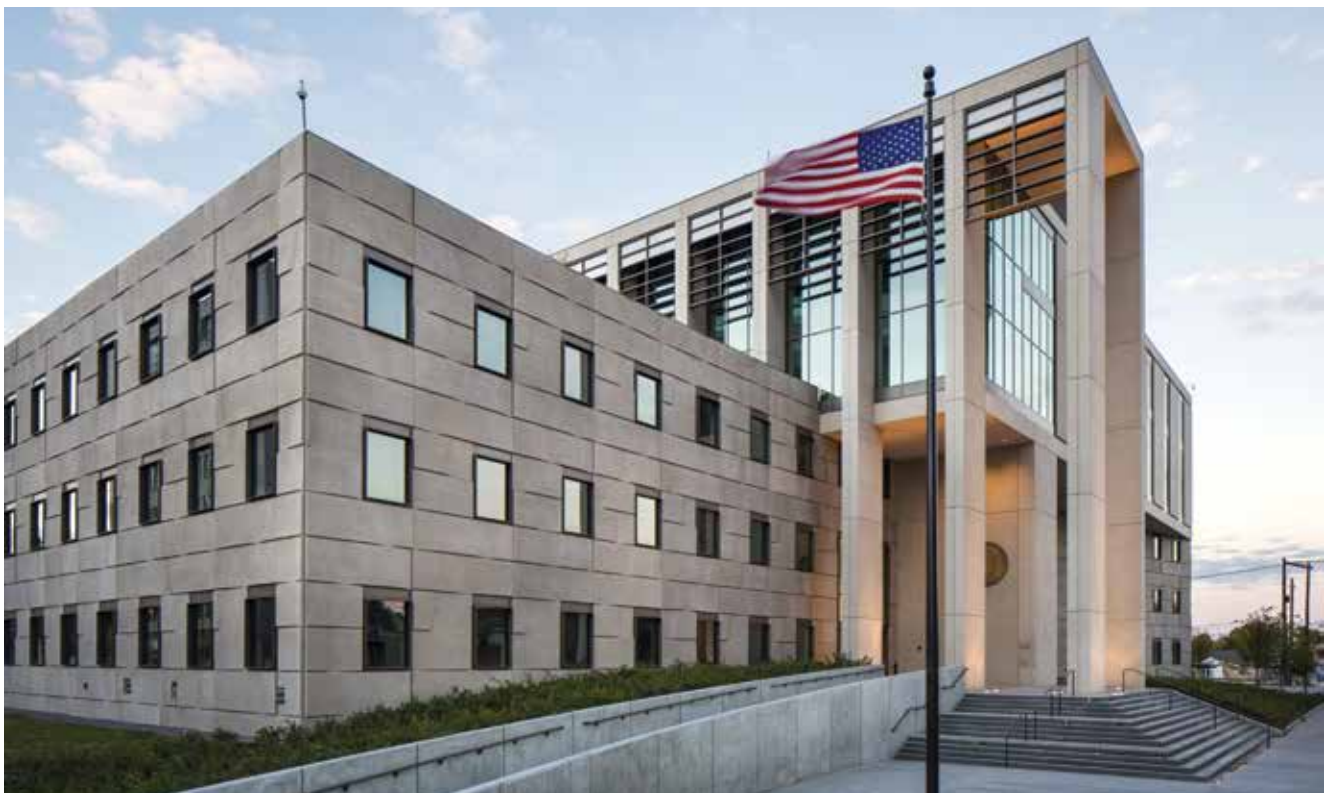
The James F. Battin United States Courthouse in Billings, Mont., features four distinct architectural elements: “visible” courtrooms with soaring windows on top, a precast concrete colonnade and portico, a base clad with architectural precast concrete panels textured to represent a solid, stone foundation, and the use of local materials throughout. All photos: Sean Airyart.
