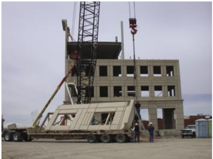
Fig. 17. Weighing 34,000 lb (15,422 kg), a 32 x 10 ft (9.8 x 3.1 m) loadbearing precast concrete wall panel is tripped from the flatbed.
