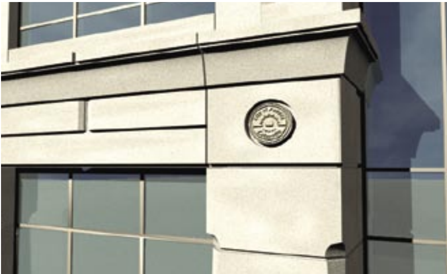
Fig. 7. Custom bronze medallions are recessed within the detailed precast panels.
