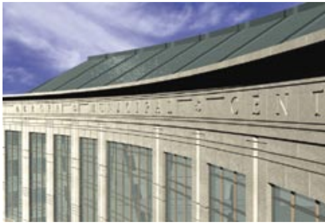
Fig. 18. Rooftop loads were reduced by using a lightweight metal enclosure around the mechanical penthouse.
