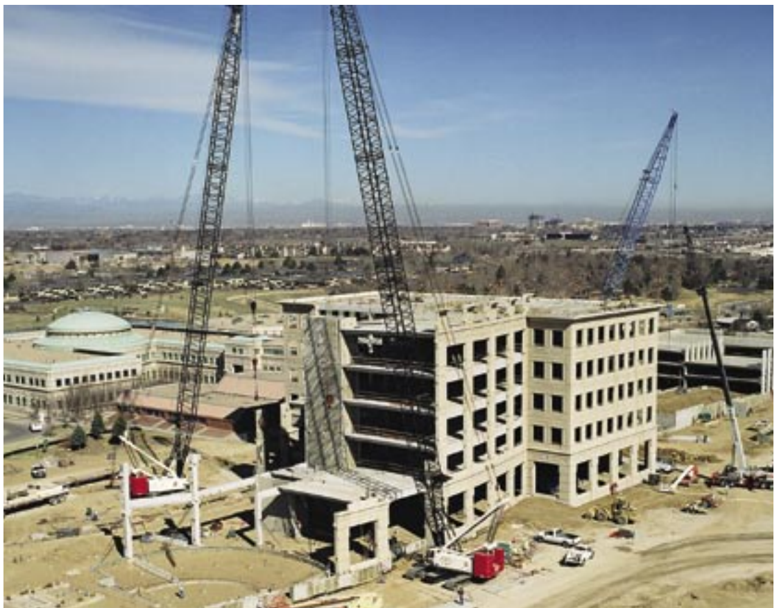
Fig. 20. Three cranes worked simultaneously towards completion of erection.
