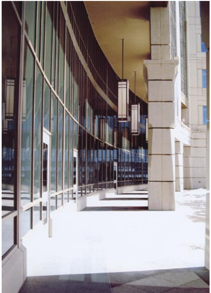
Fig. 12. An elegant loggia with free-standing precast concrete columns greets visitors to the complex.
